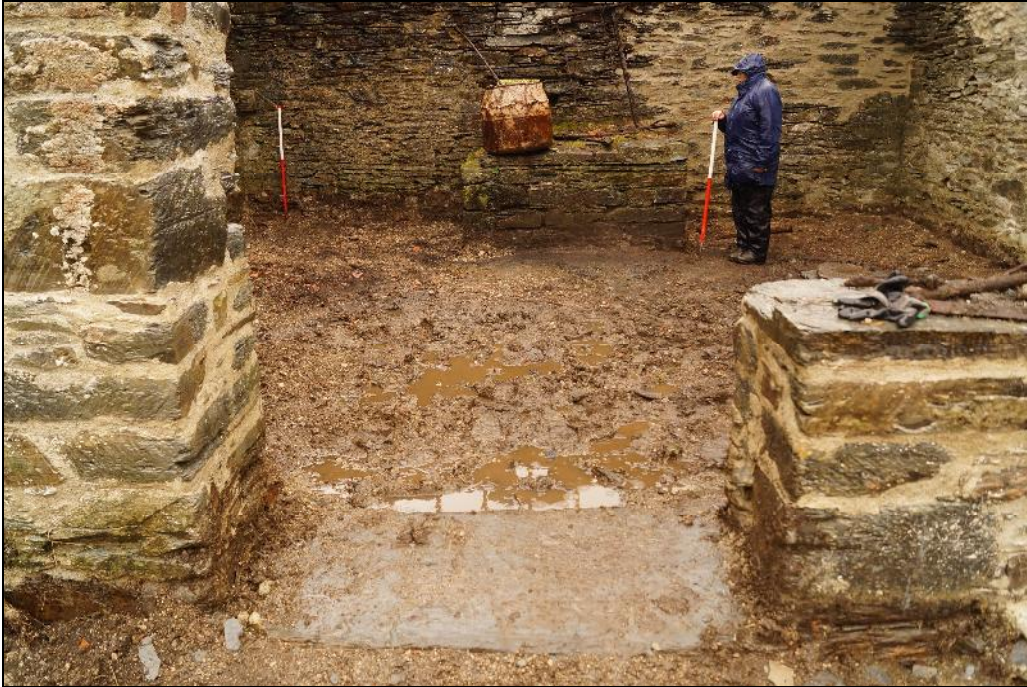
Plate 29: CEM2017_129. A view of the entrance into Room A, the forge, showing the threshold stone (004), after the removal of the layers (001) and (002) inside the room. This level was maintained and terram and gravel was to be laid across the interior without further material being removed. Looking north-northwest.
