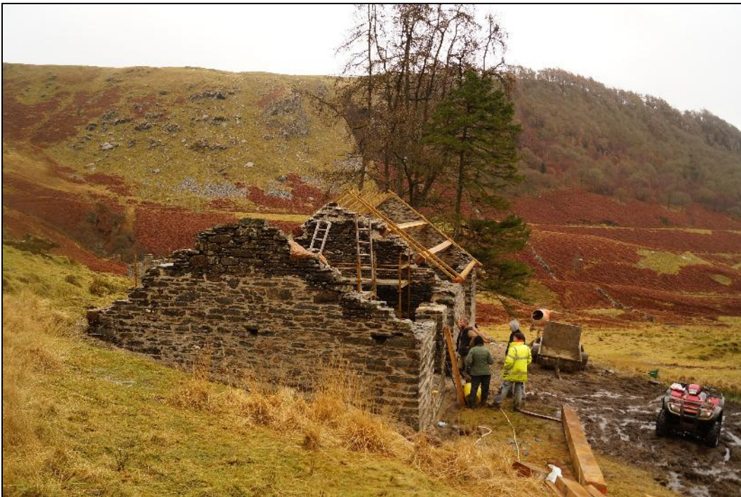
Plate 6: CEM2017_106. A view of the former mine smithy building. Looking east-northeast.
