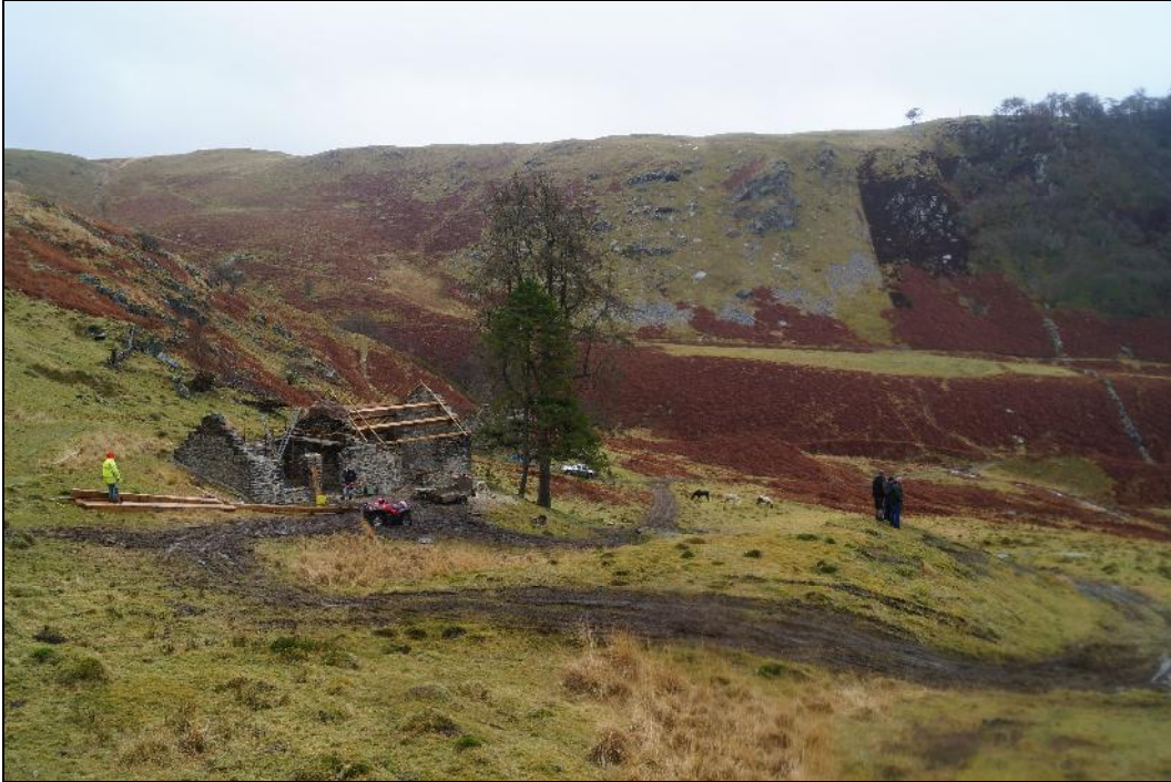
Plate 1: CEM2017_101. A general view of the former mine smithy building. It stands on the same site as the earlier Pen y Gwaith cottage and may incorporate some fabric of the dwelling. Looking north-northeast.
