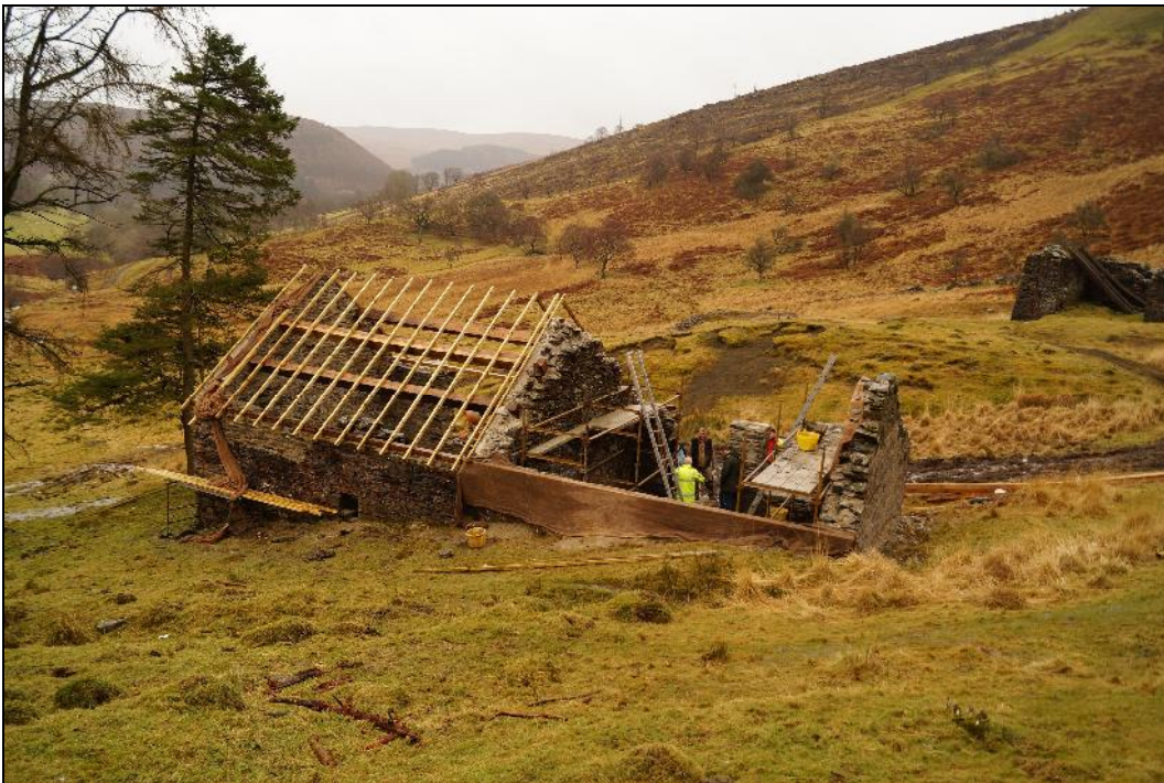
Plate 4: CEM2017_104. A view of the former mine smithy building. Looking south-southeast.
