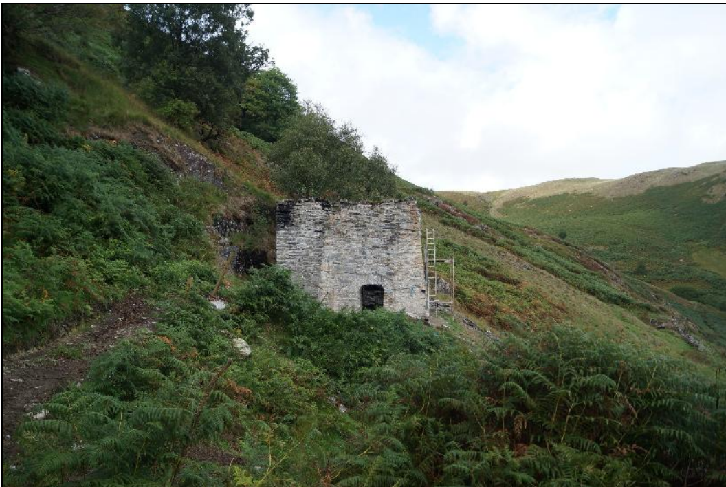
Plate 18: CEM2018_125 A view of the wheel pit. Looking north-northeast.
