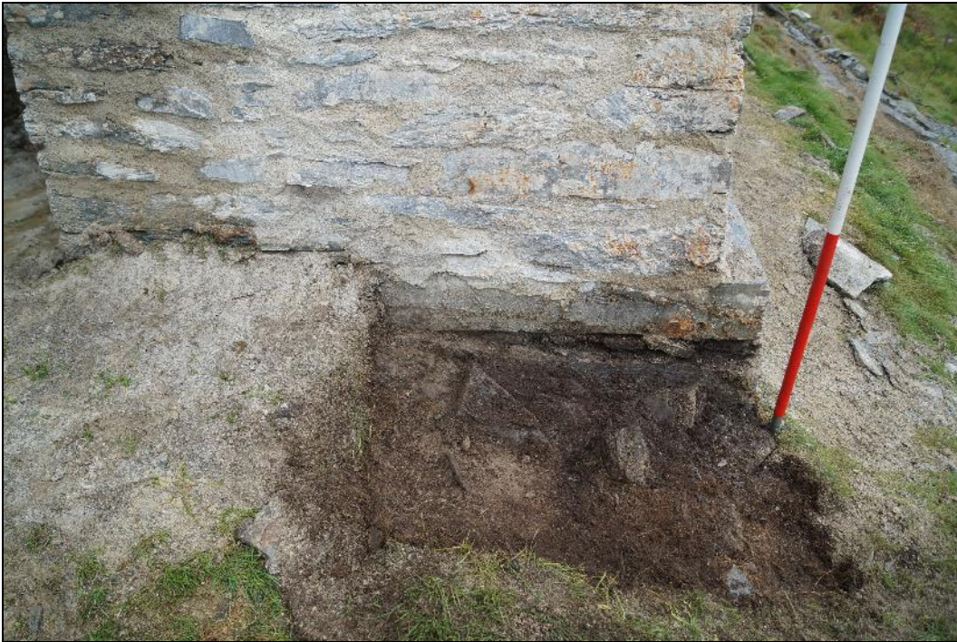
Plate 7: CEM2018_107. A view of test pit after the removal of the turf layer (001). The rubble (002) associated with the gradual dereliction of the wheel pit is revealed. Looking north-northeast.
