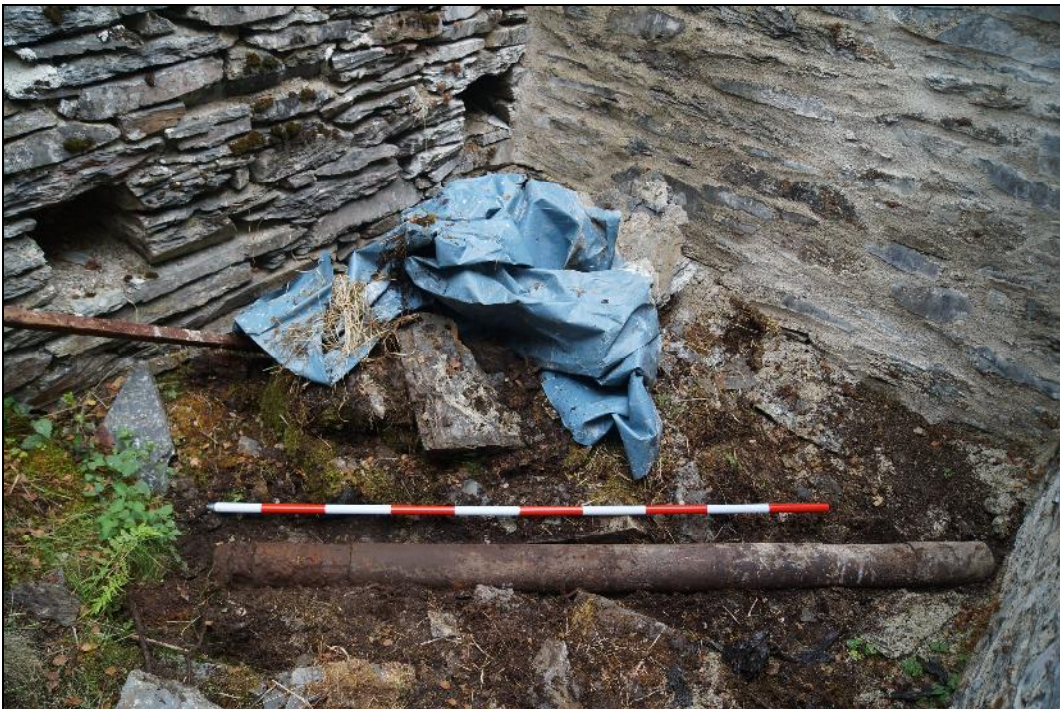
Plate 14: CEM2018_121. A view of the iron axle that is now laying in a cell to the west of the wheel pit. Looking east.
