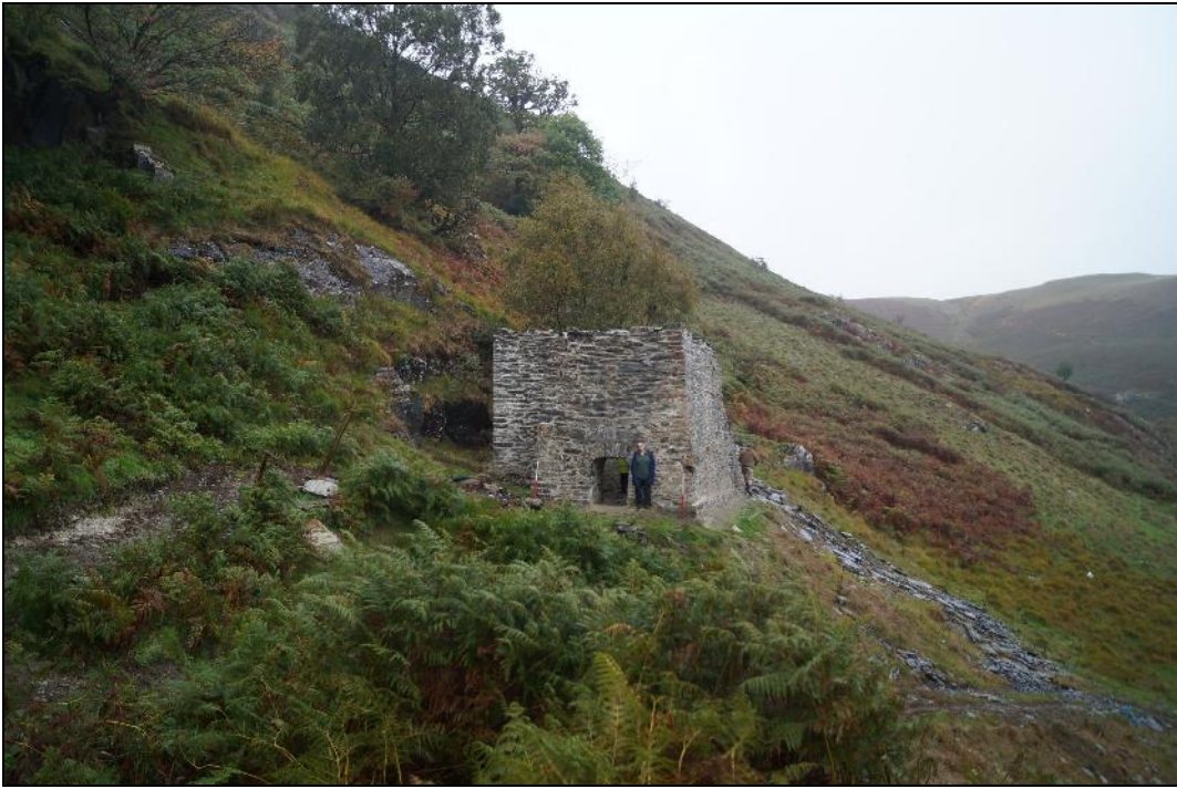
Plate 20: CEM2018_127. A view of the wheel pit. Looking north-northeast.
