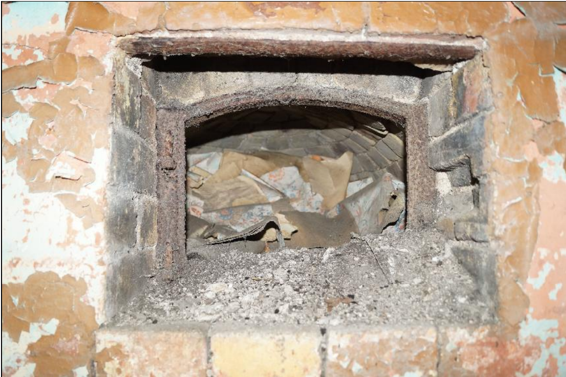
Plate 36: CYB2018_036. A view into the bread oven in Room 02 showing the cast iron door frame and the firebrick lining inside the oven. Looking south-southeast.
