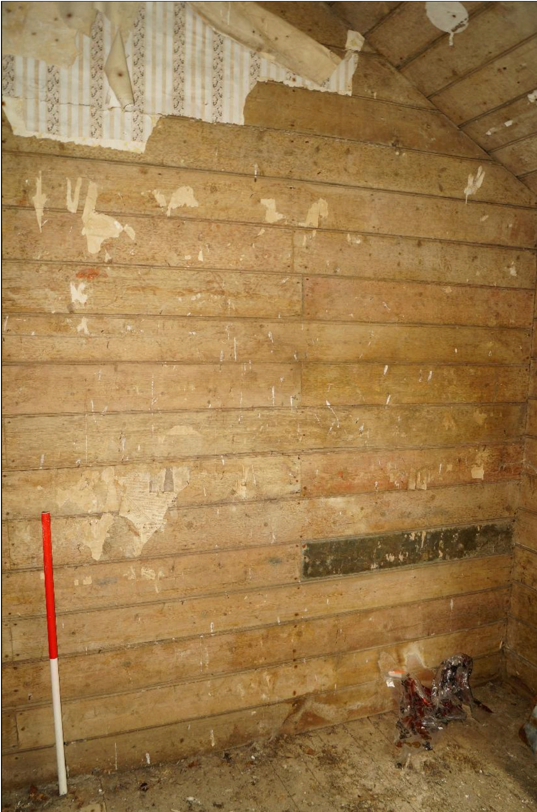
Plate 70: CYB2018_070. A view of the western side of Room 05. Looking northwest.
