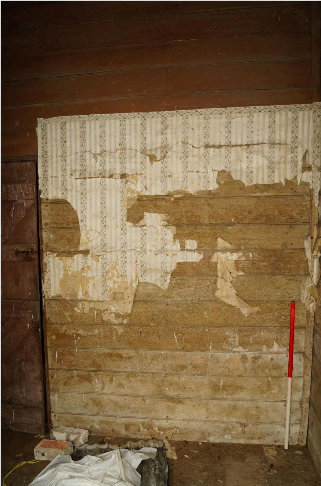
Plate 78: CYB2018_078. A view of the southern side of Room 06, showing surviving wallpaper and newspaper lining. Looking south-southwest.
