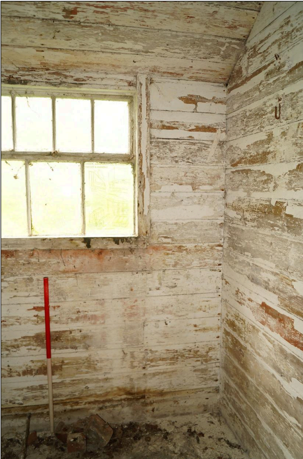
Plate 60: CYB2018_060, A view inside Room 04. Looking north-northeast.
