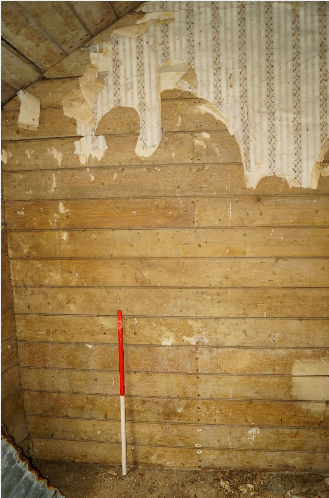
Plate 74: CYB2018_074. A view of the eastern side of Room 05. Looking east-southeast.
