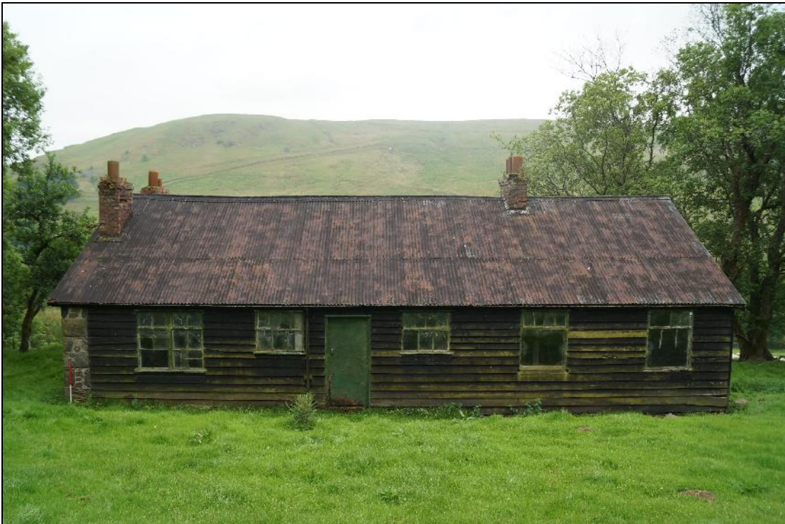
Plate 9: CYB2018_009. A view of the rear of the Dam Builders' Hut. Looking south-southwest.
