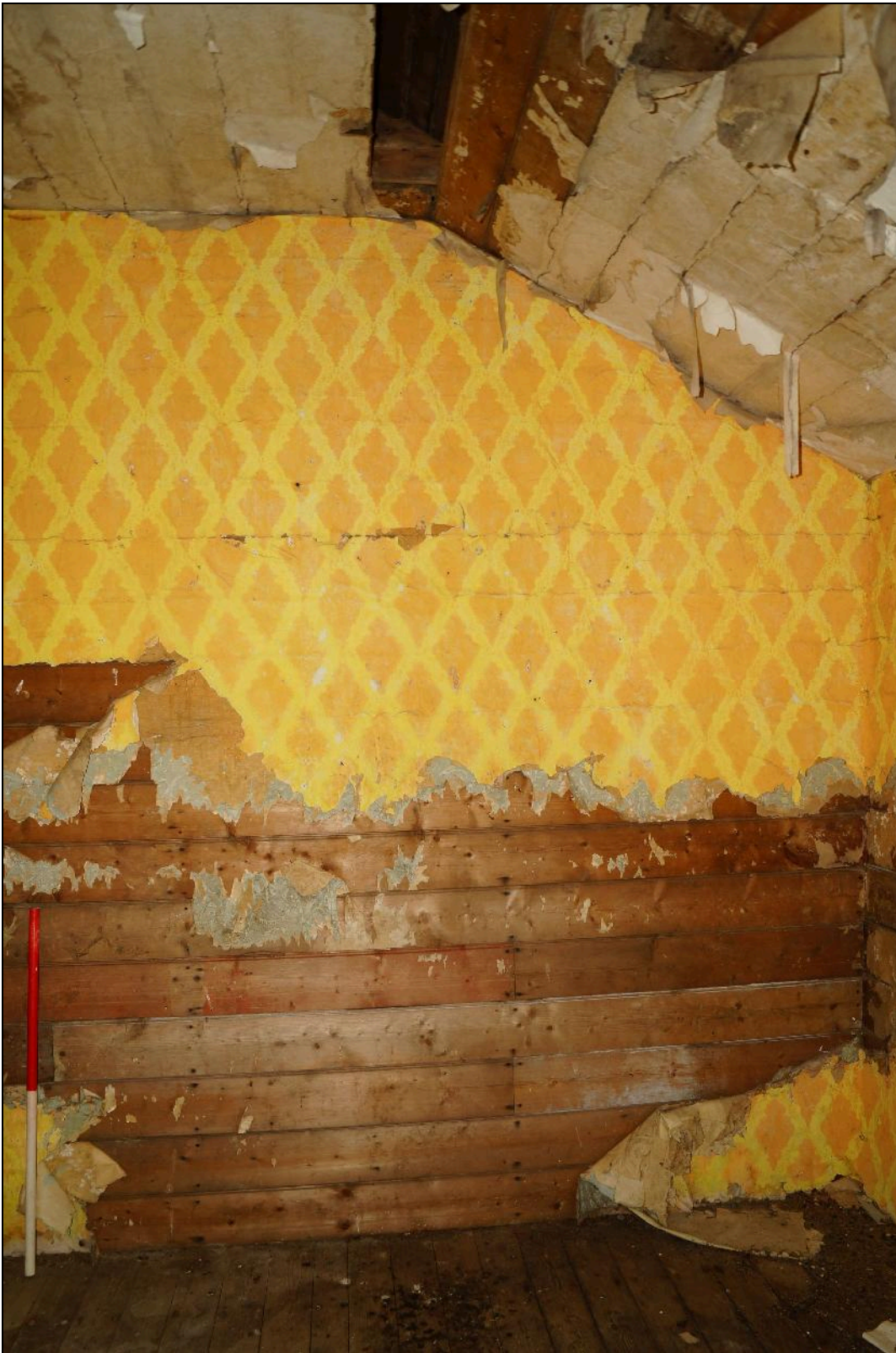
Plate 104: CYB2018_104. A view of the eastern side of Room 09. Looking southeast.
