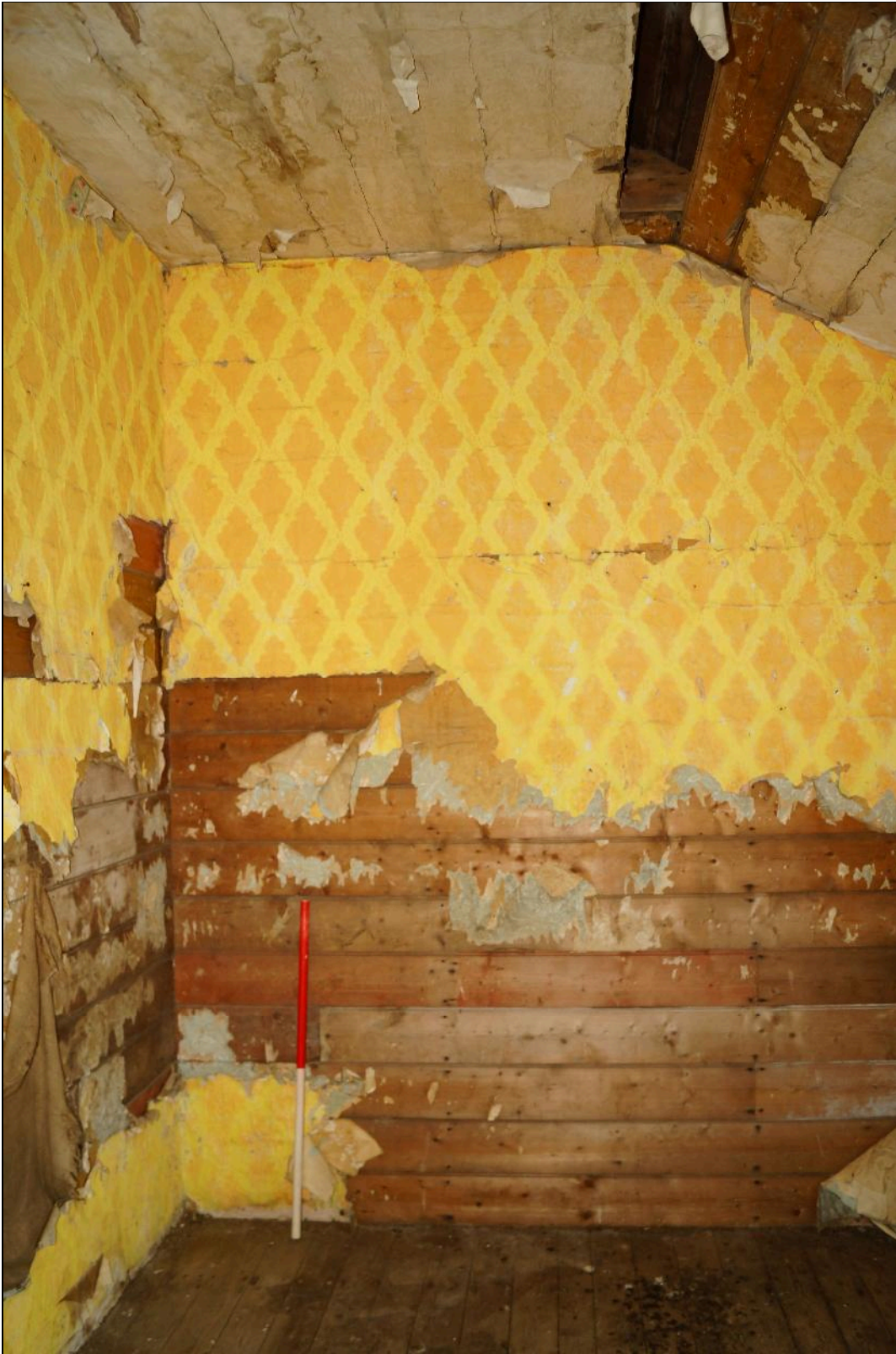
Plate 103: CYB2018_103. A view of the eastern side of Room 09. Looking east-southeast.
