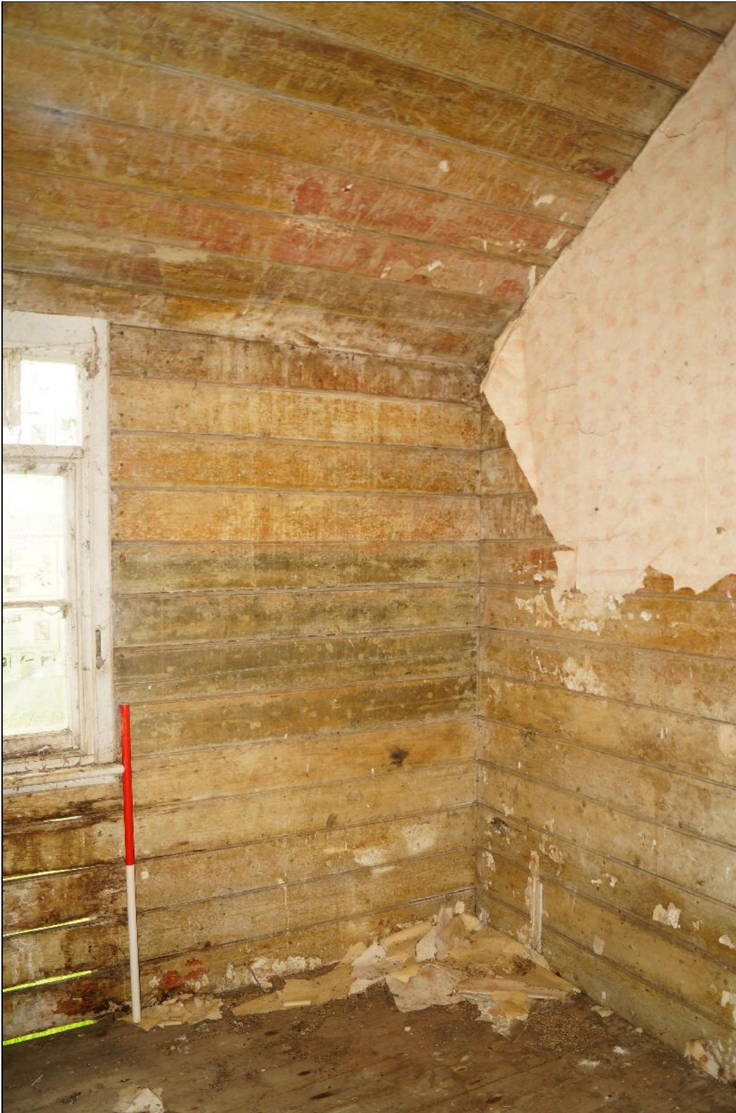
Plate 97: CYB2018_097. A view of the southern side of Room 08. Looking southwest.
