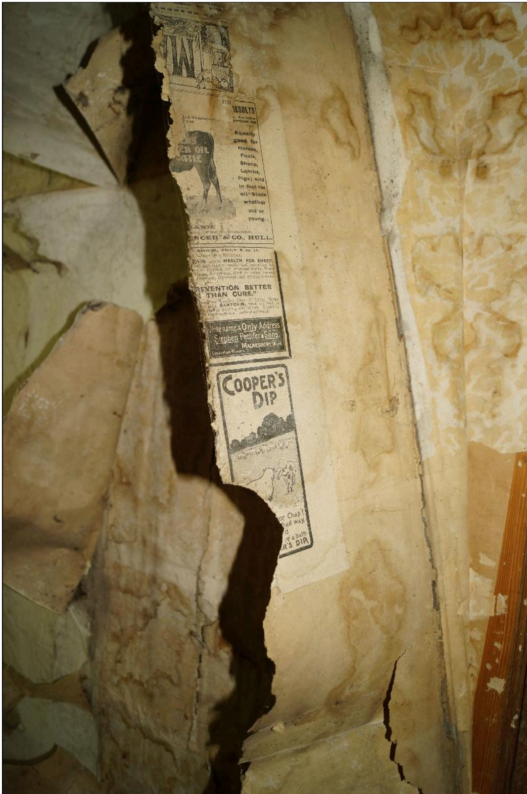
Plate 110: CYB2018_110. A view of exposed newspaper lining in the ceiling of Room 09. Looking north-northeast.
