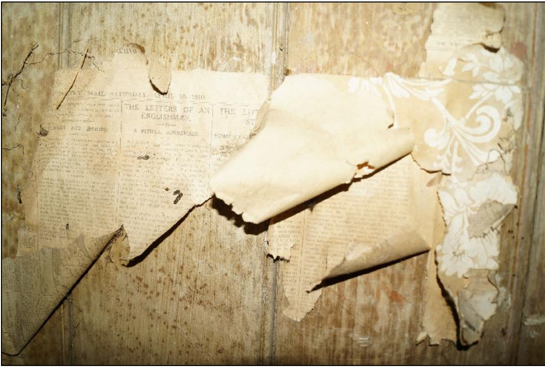
Plate 77: CYB2018_077. A view of exposed newspaper lining on the southern wall of Room 06, showing a fragment from the Daily Mail of Saturday, April 16, 1910. Looking south-southwest.
