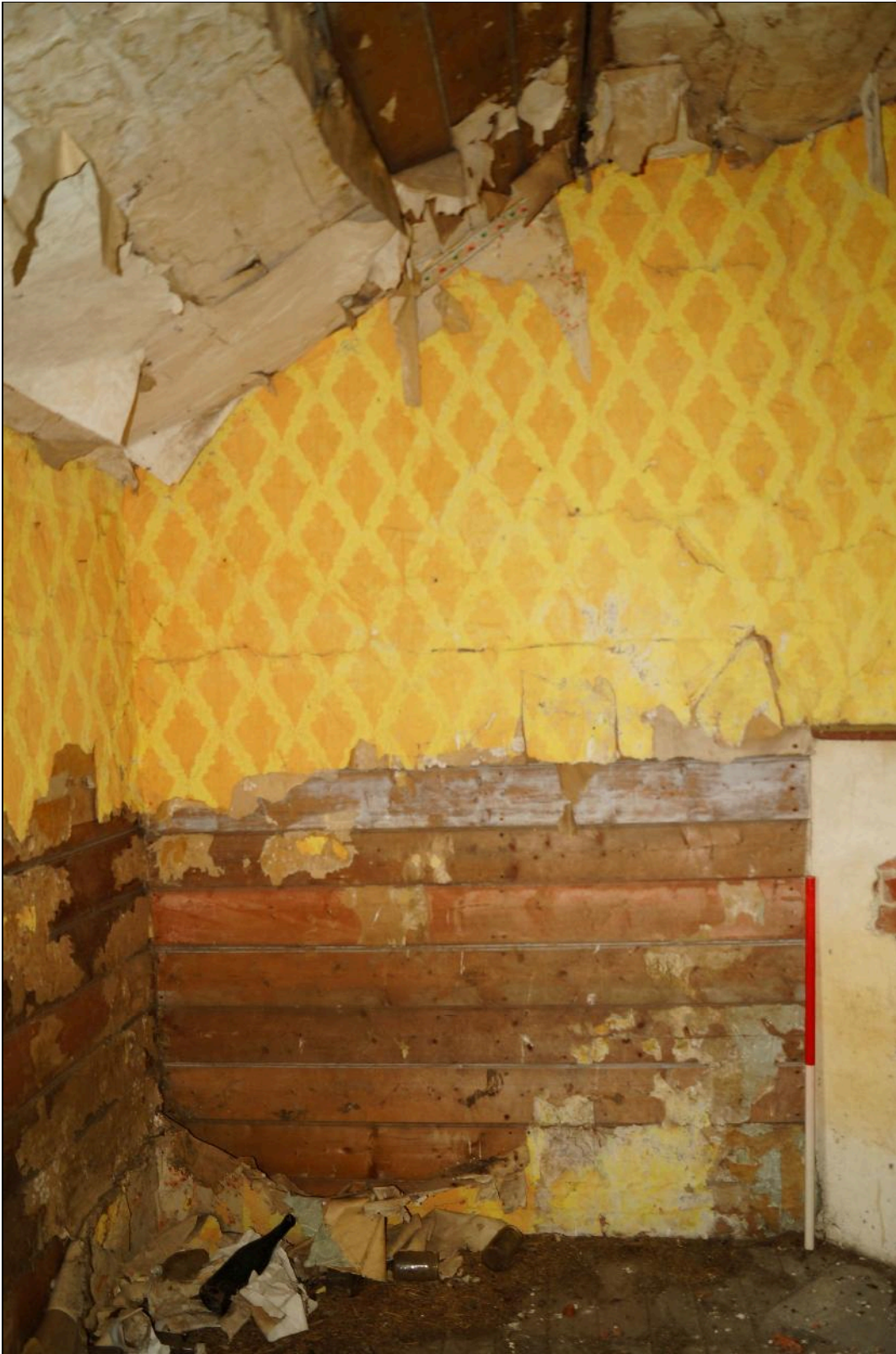
Plate 100: CYB2018_100. A view of the western side of Room 09. Looking west-northwest.
