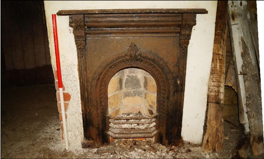
Plate 65: BTC2017_065. Another view of the fireplace in the southern side of Room 05. Note the red-brick chimney breast exposed to the left. Looking south-southwest.
