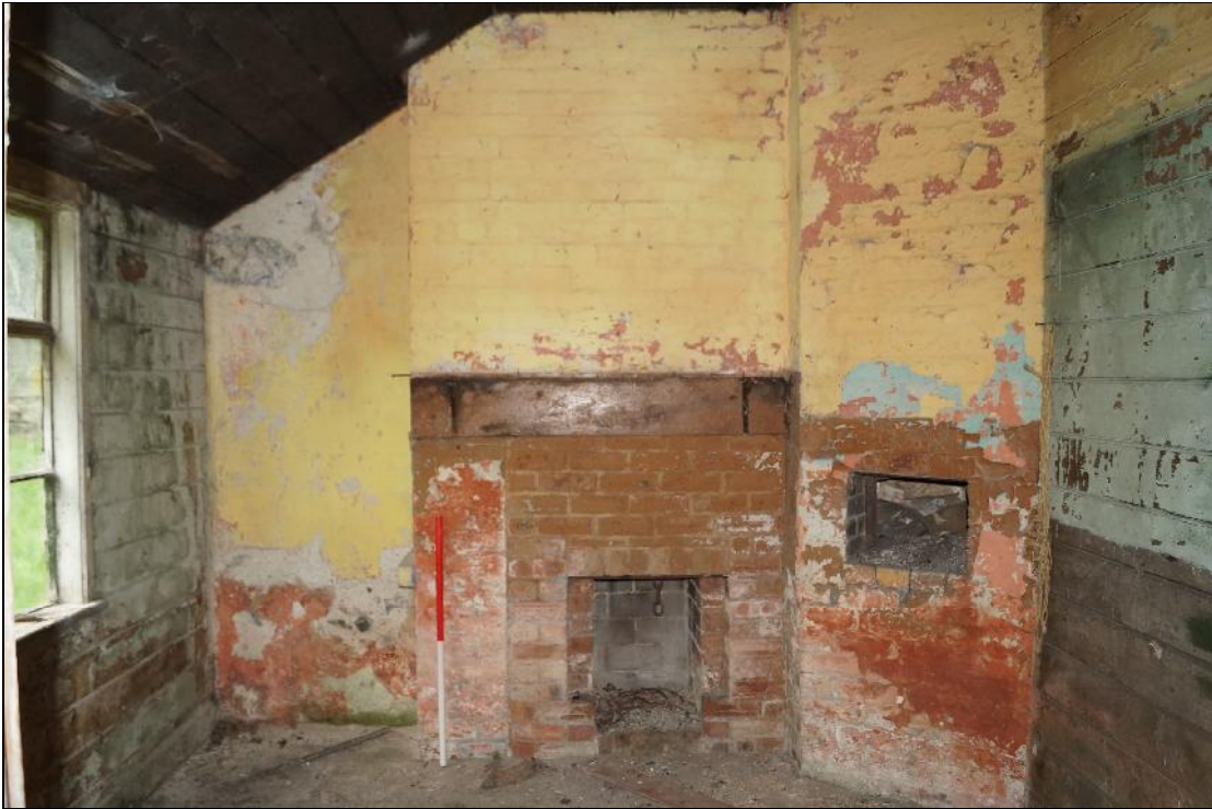
Plate 33: CYB2018_033. A view of the fireplace and oven in Room 02. Note the brick walling of the chimney breast. Looking east-southeast.
