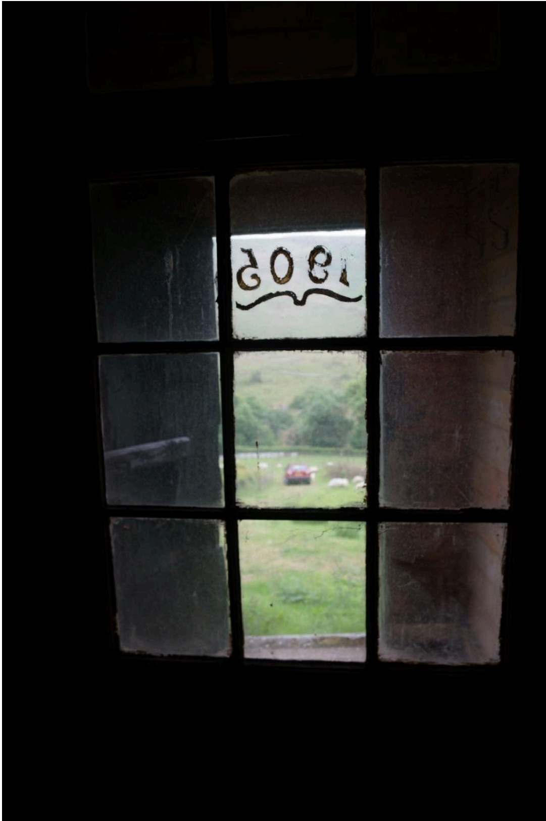
Plate 20: CYB2018_020. A view through the glass panes of the front door. Looking south-southwest.
