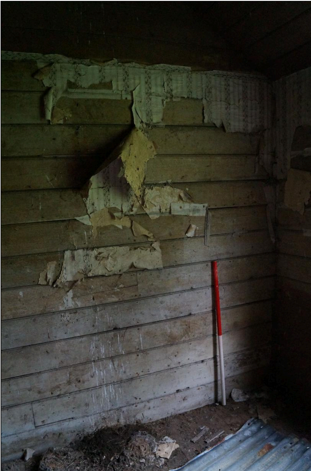
Plate 83: CYB2018_083. A view of the western side of Room 06. Note the wooden flooring. Looking northwest.
