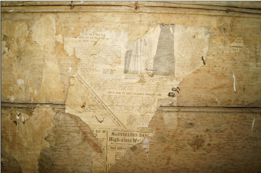
Plate 68: CYB2018_068. A view of newspaper lining the western wall of Room 05. Looking west-northwest.
