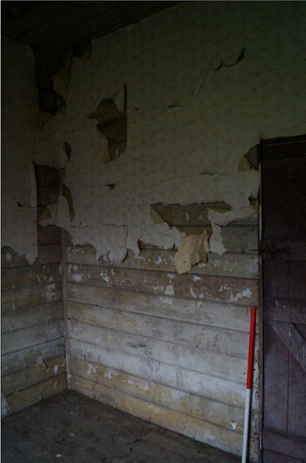
Plate 95: CYB2018_095. A view of the northern side of Room 08. Looking north-northwest.
