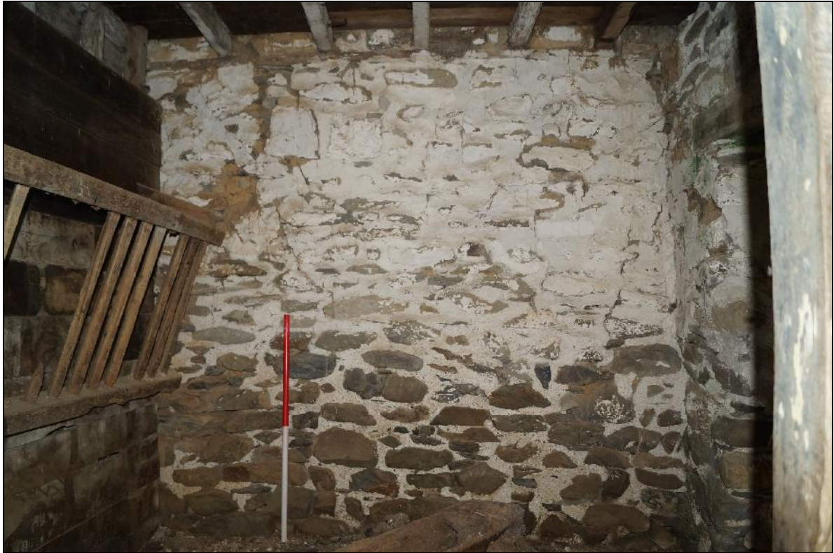
Plate 69: CYD2018_069, the northern wall of the "dairy", looking north-northwest.
