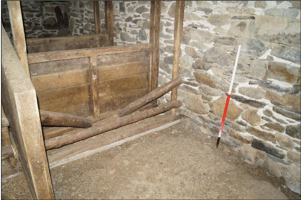
Plate 49: CYD2018_049, internal view of the cowshed, showing the western feeding stall at the northern end of the cowshed, looking south.
