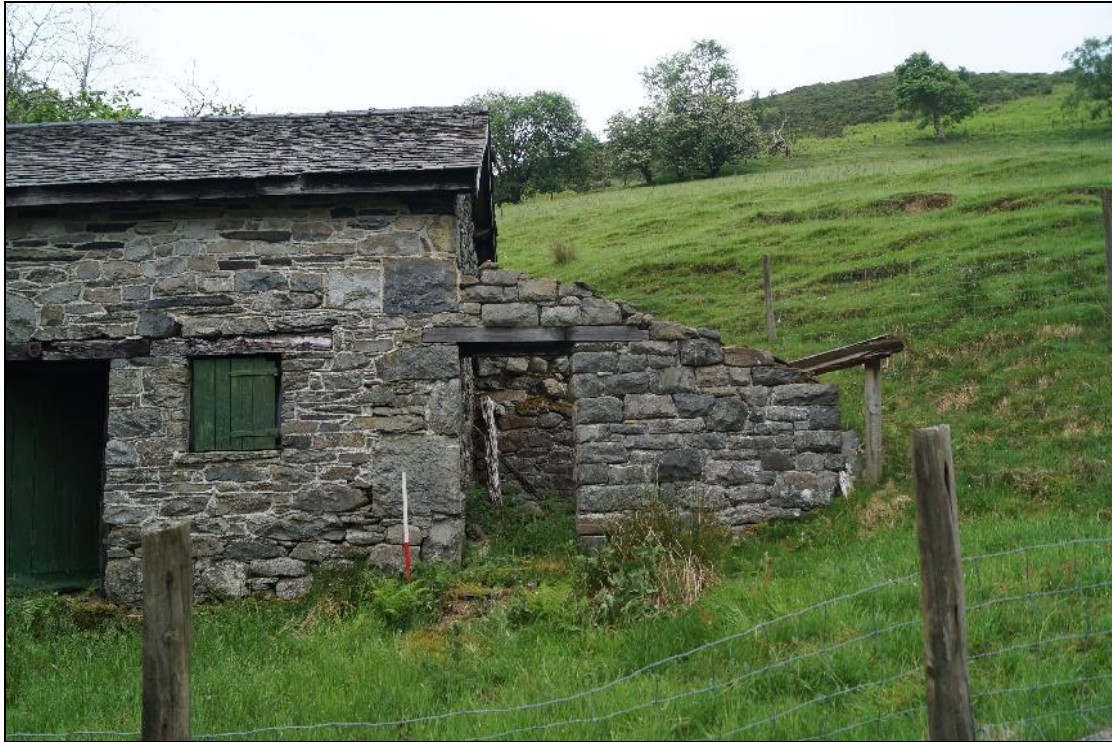
Plate 3: CYD2018_003, external view of the now roofless lean-to extension at the southern end of the stable looking east-northeast.
