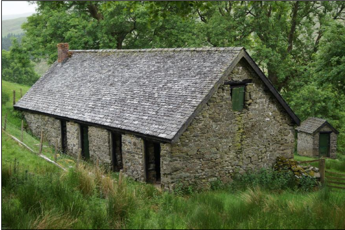
Plate 13: CYD2018_013, external view of the house and cowshed building looking southwest.
