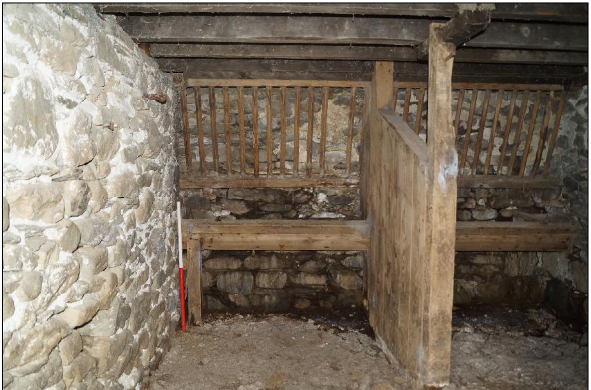
Plate 22: CYD2018_022, an internal view of the stable, showing the northern feeding stall, looking east-northeast.
