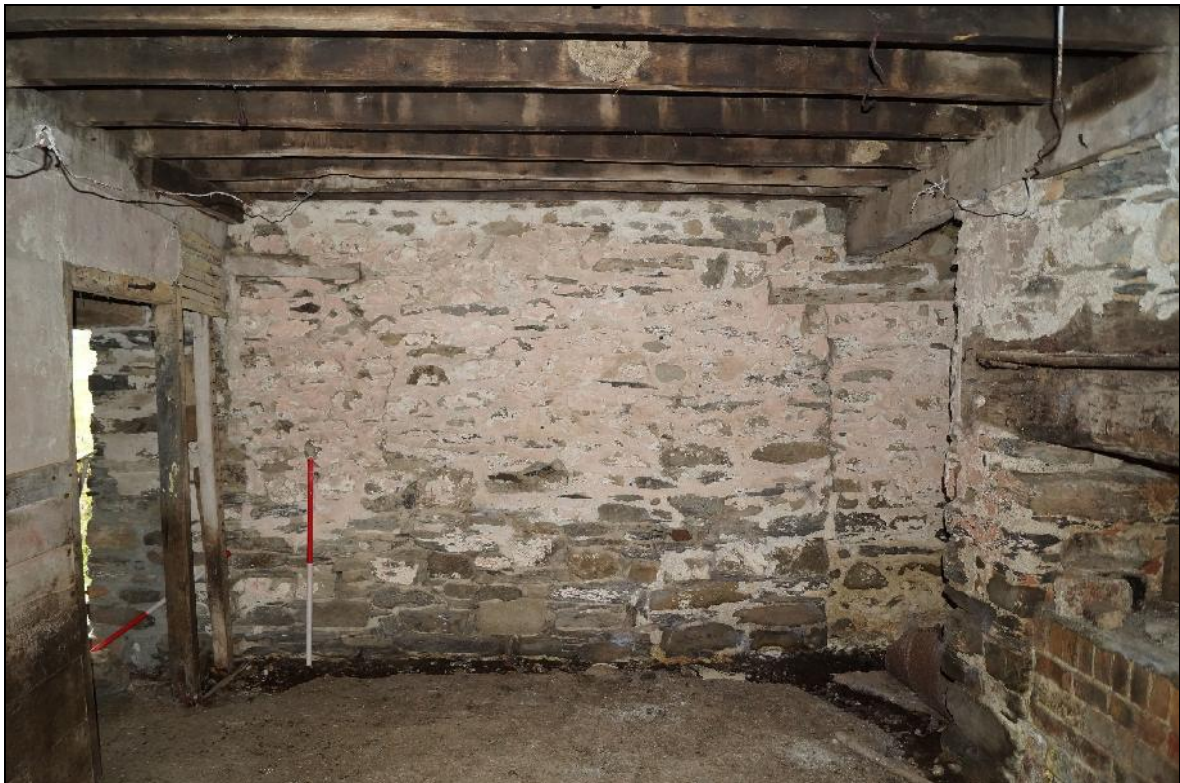
Plate 90: CYD2018_090, an interior view of the eastern wall of the kitchen, looking east-northeast, showing an apparent blocked up doorway to the right-hand side.
