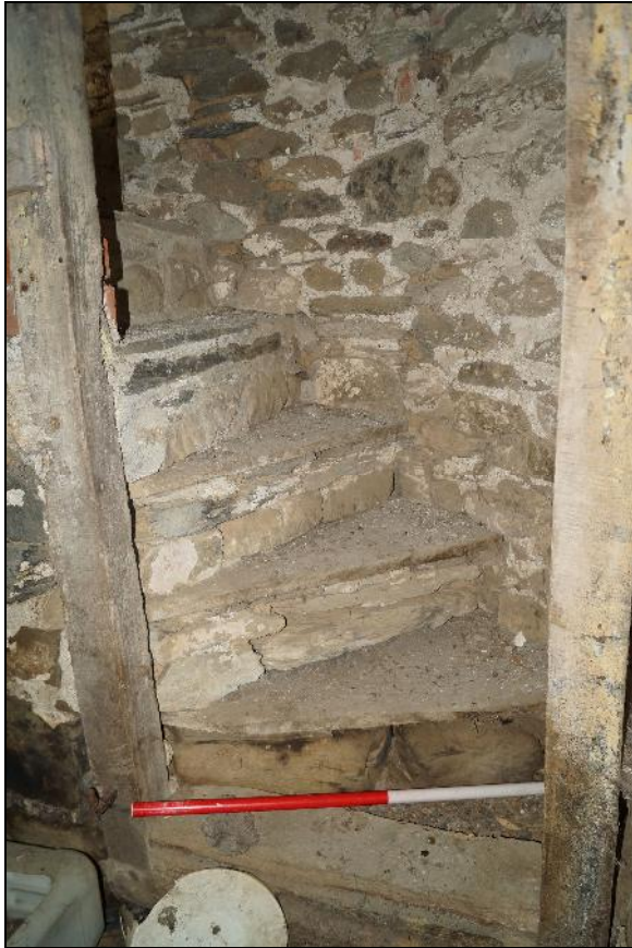
Plate 101: CYD2018_101, a view of the stone steps of the stairs to the loft above the kitchen, looking southeast.
