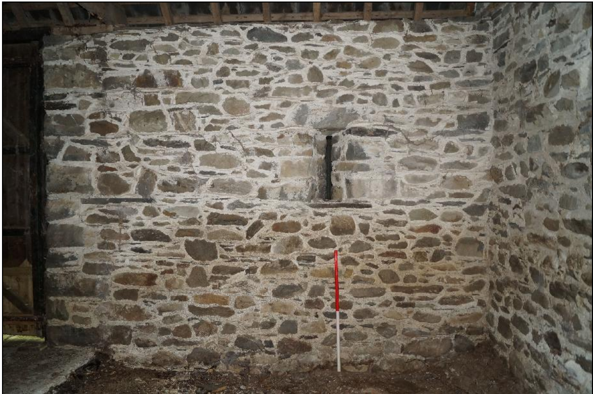
Plate 130: CYD2018_130, an interior view of the barn, looking east towards the southern end of the west wall, where a blocked-up slit window can be seen.
