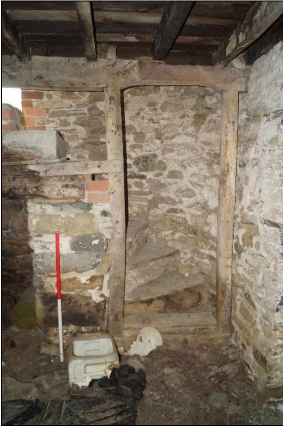
Plate 97: CYD2018_097, the stone steps of the stairs to the loft which are in the southwestern corner of the kitchen, looking south-southeast.
