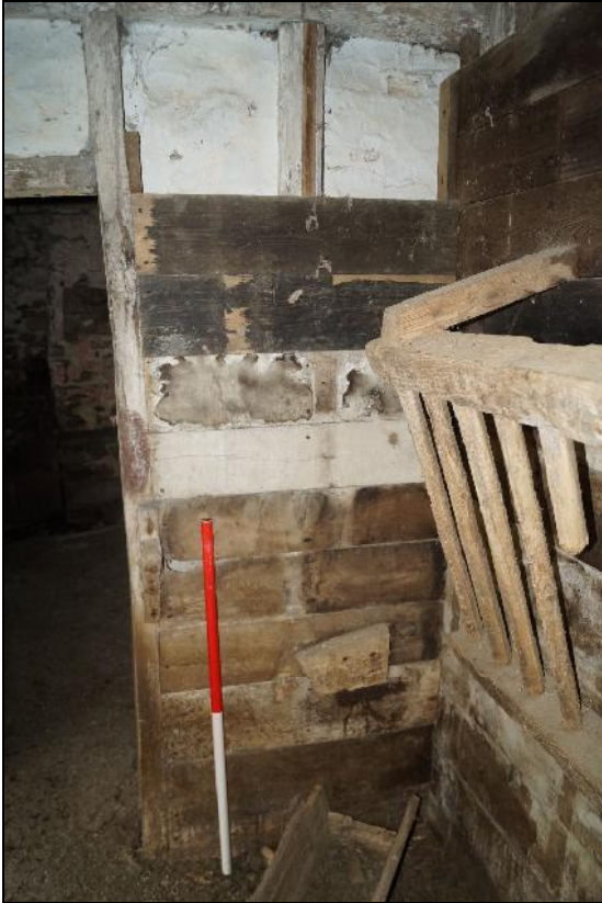
Plate 73: CYD2018_073, the southern wall of the "dairy", looking south-southeast. Note the timber framing and lath and plaster partitioning at the top, with horizontal planking below.
