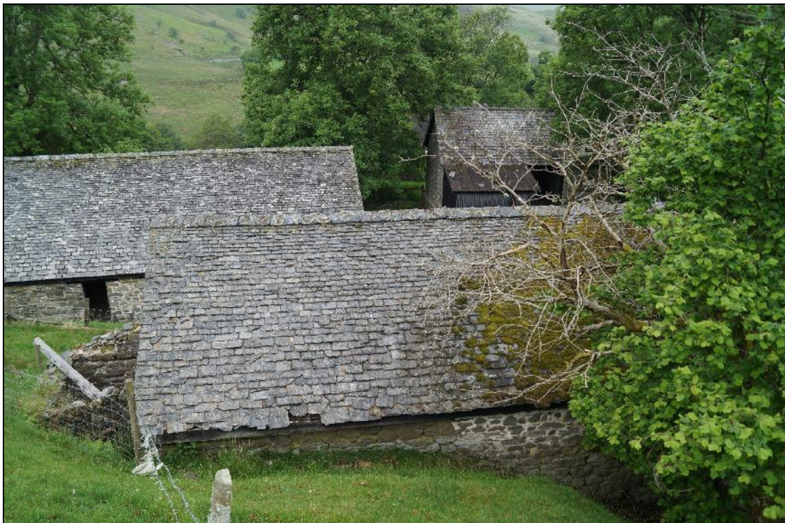
Plate 8: CYD2018_008, external view of the stable and cartshed roof looking west-southwest.
