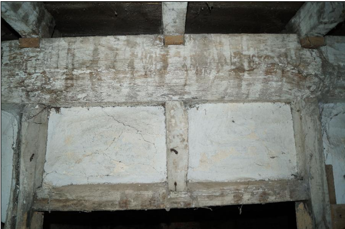
Plate 75: CYD2018_075, the doorway in the southern wall of the "dairy", leading into the kitchen, looking south-southwest, showing the timber framing and lath and plaster partitioning.
