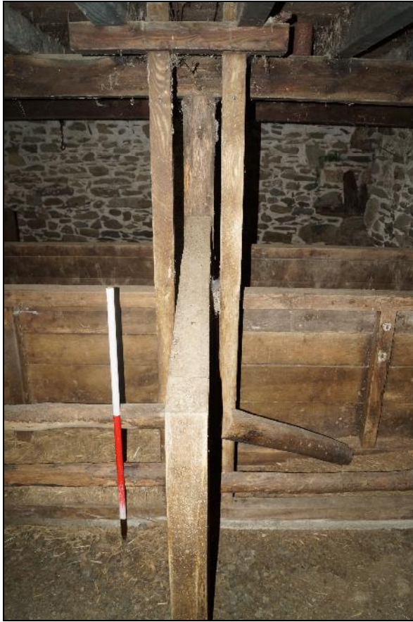
Plate 51: CYD2018_051, internal view of the cowshed, showing the turned posts between the central and western feeding stalls at the northern end of the cowshed, looking south.
