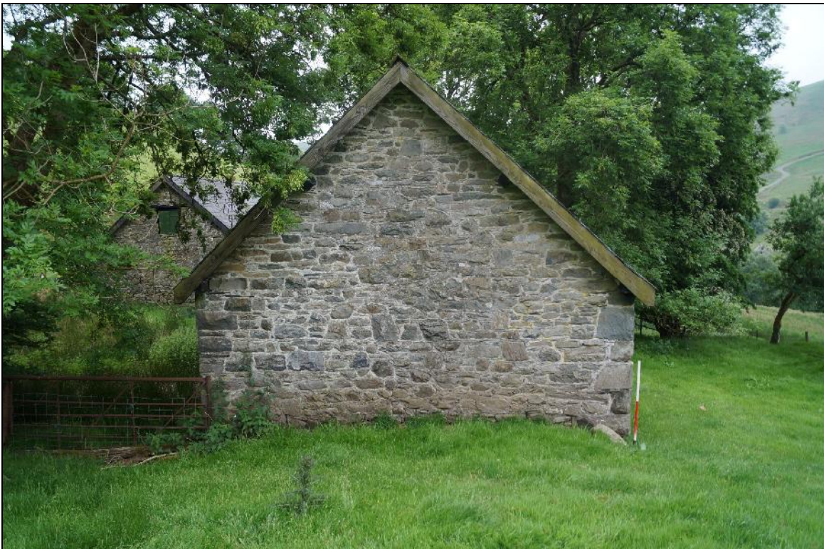
Plate 118: CYD2018_118, an external view of the northern gable wall of the barn at Cwmclyd, looking south.
