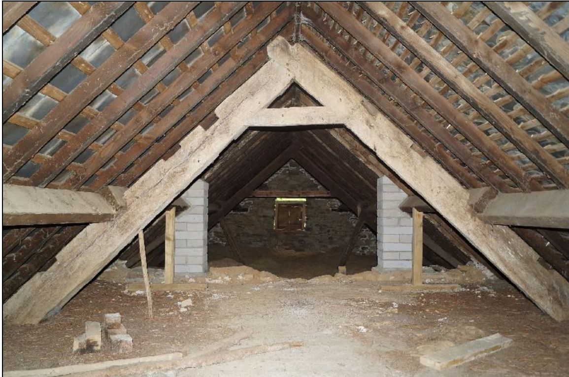
Plate 105: CYD2018_105, a view into the loft of Cwmclyd house and cowshed, showing a modern roof with one original roof truss in place, looking north-northwest.
