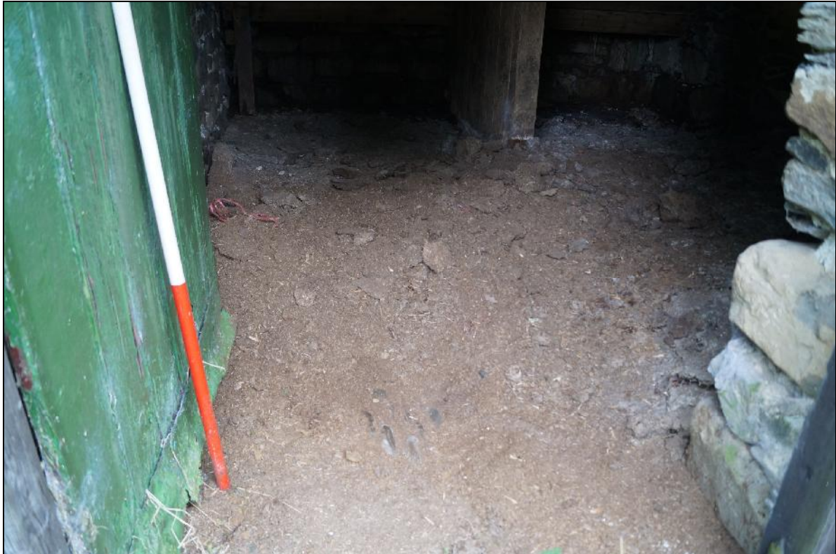
Plate 35: CYD2018_035, a view through the doorway into the stable, with evidence of a cobbled floor exposed through the accumulated debris, looking east-northeast.
