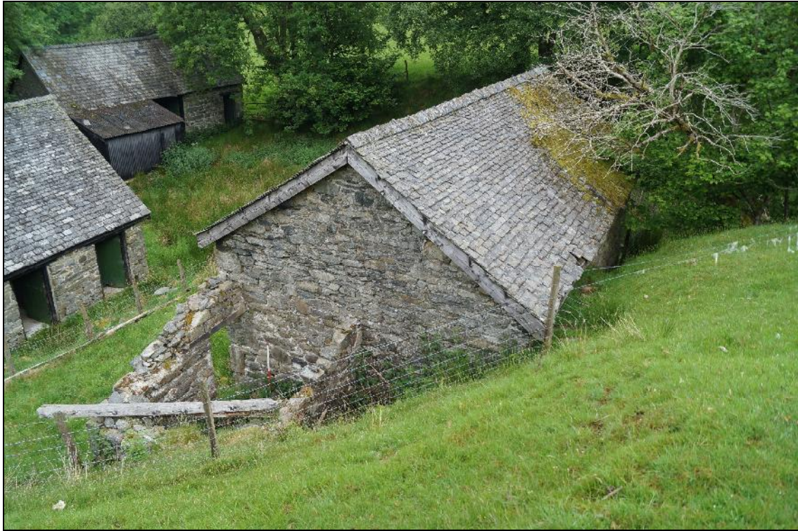
Plate 7: CYD2018_007, external view of the stable and cartshed building looking northwest.
