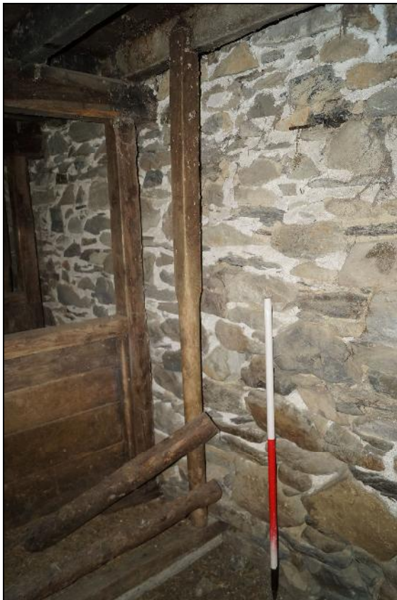
Plate 50: CYD2018_050, internal view of the cowshed, showing a turned post in the western feeding stall at the northern end of the cowshed, looking south.
