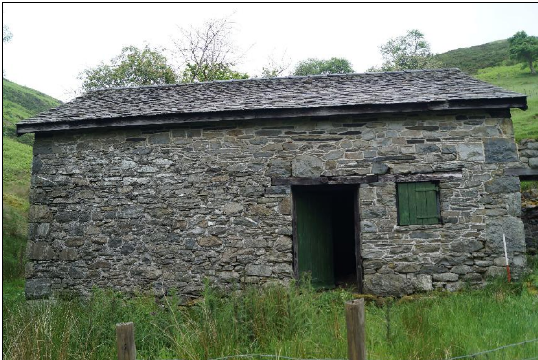
Plate 2: CYD2018_002, external view of the stable and cartshed building, looking east-northeast.
