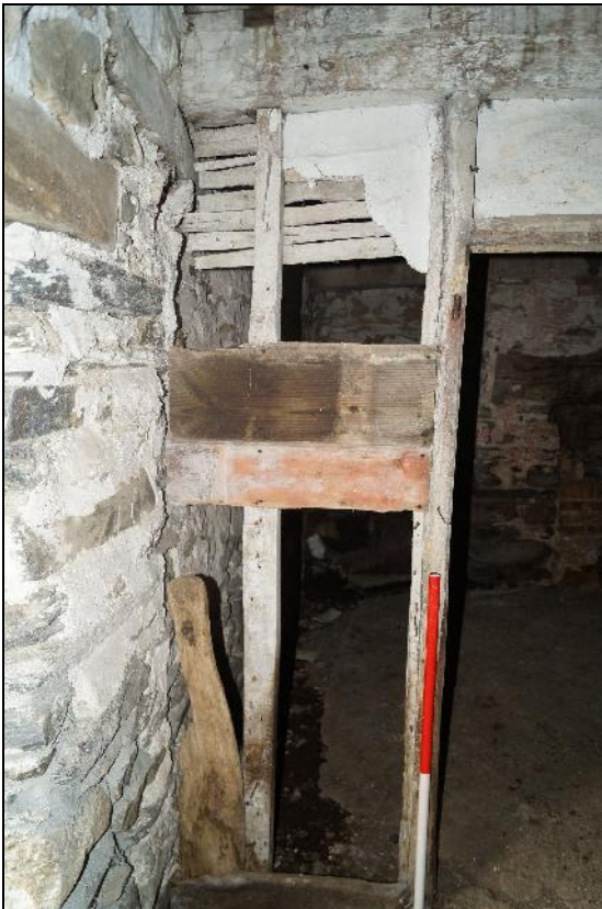
Plate 73: CYD2018_073, the southern wall of the "dairy", looking south-southeast. Note the timber framing and lath and plaster partitioning at the top, with horizontal planking below.
