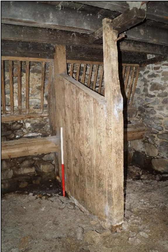
Plate 26: CYD2018_026, an internal view of the stable, showing the partition between the two feeding stalls, looking east-southeast.
