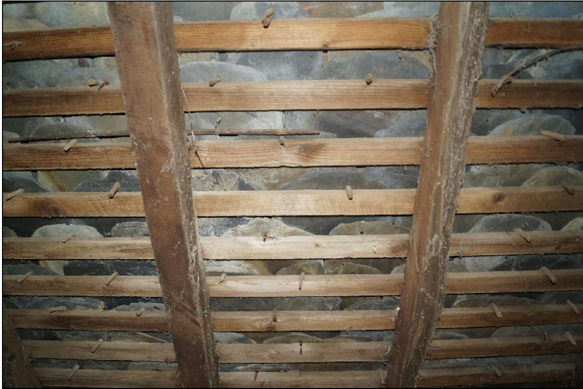
Plate 107: CYD2018_107, a view of the modern roof from inside the loft, showing modern timberwork supporting original slates which have been fixed using wooden pegs, looking east-northeast.
