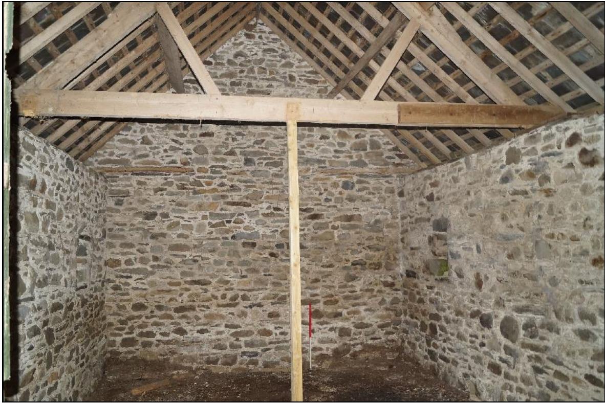
Plate 123: CYD2018_123, an interior view of the barn, looking south towards the gable wall. Note the modern roof and supporting timbers.
