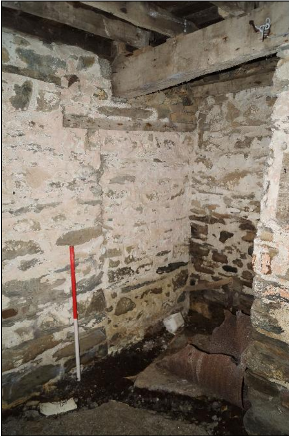
Plate 91: CYD2018_091, an interior view of the southern end of the eastern wall of the kitchen, looking southeast, showing an apparent blocked up doorway.
