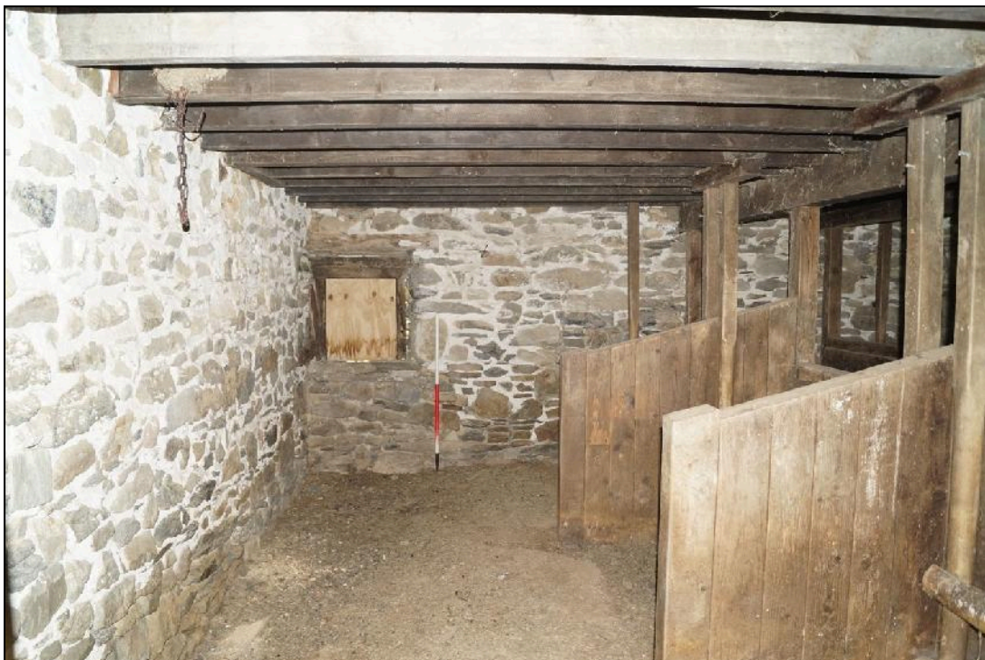
Plate 56: CYD2018_056, internal view of the cowshed, showing the feeding stalls at the southern end of the cowshed and looking west-southwest. A pitching door is seen on the far wall.
