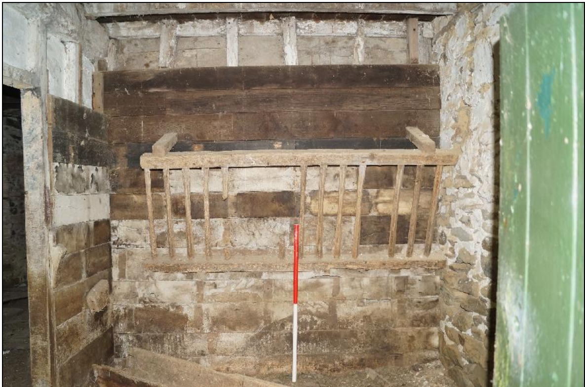
Plate 68: CYD2018_068, A feeding stall in the "dairy" (according to the RCAHMW's 1988 survey) of the house at Cwmclyd, looking south-southwest.
