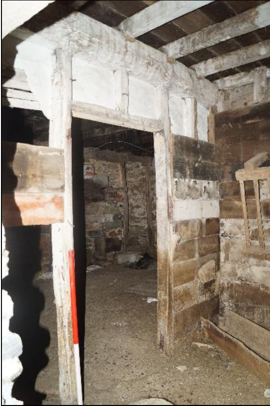
Plate 75: CYD2018_075, the doorway in the southern wall of the "dairy", leading into the kitchen, looking south-southwest, showing the timber framing and lath and plaster partitioning.
