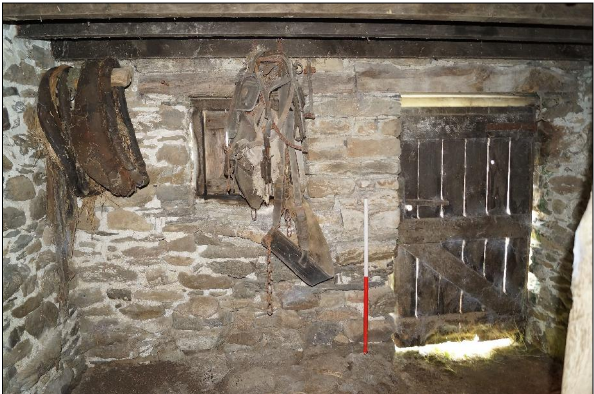
Plate 30: CYD2018_030, an internal view of the stable, showing the western wall, window and doorway, looking west-southwest.
