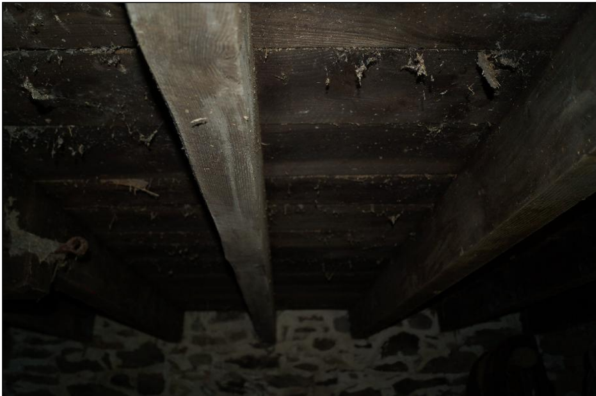
Plate 34: CYD2018_034, the ceiling of the stable is composed of modern, machine-sawn beams with a modern plank floor above. The original beams and flooring must have been replaced in modern times.
