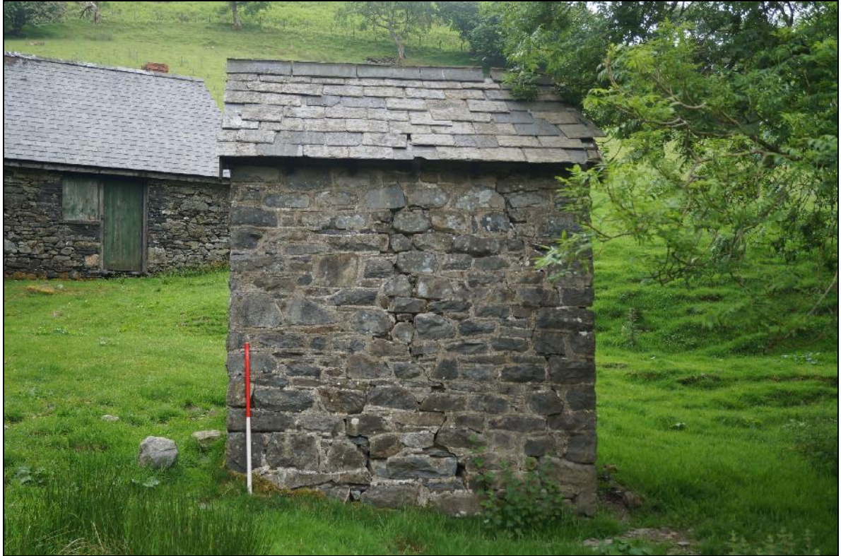
Plate 111: CYD2018_111, a view of the privy at Cwmclyd, looking east-southeast.
