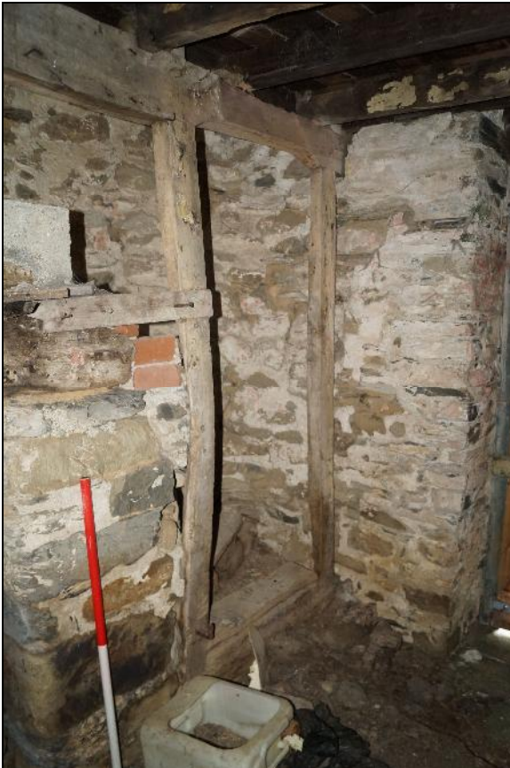
Plate 98: CYD2018_098, the stone steps of the stairs to the loft which are in the southwestern corner of the kitchen, looking southwest.
