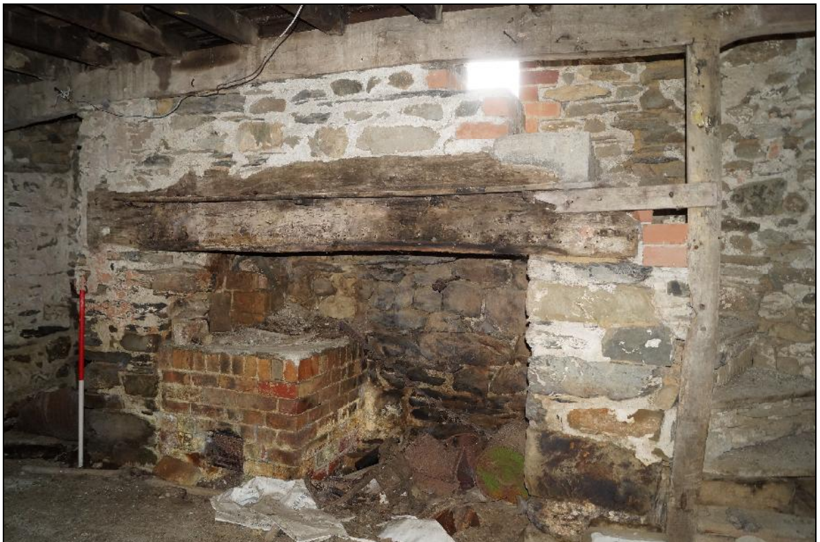
Plate 94: CYD2018_094, an interior view of the fireplace in the kitchen, looking southeast. The brick insert was the housing for a water boiler.
