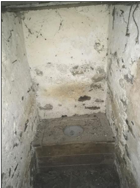
Plate 114: CYD2018_114, an interior view of the privy at Cwmclyd, showing the original toilet still in place, looking south-southwest.
