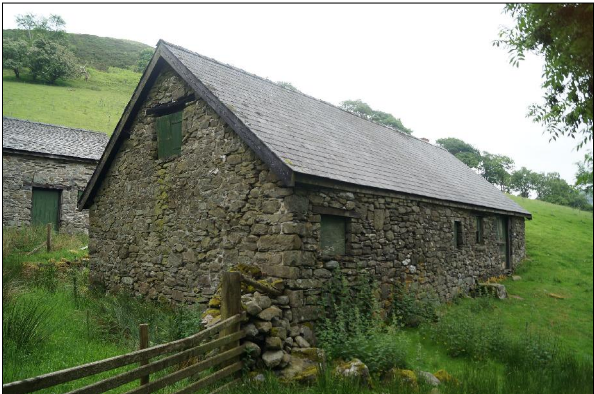
Plate 116: CYD2018_116, an external view of the cowshed and house at Cwmclyd, looking southeast.
