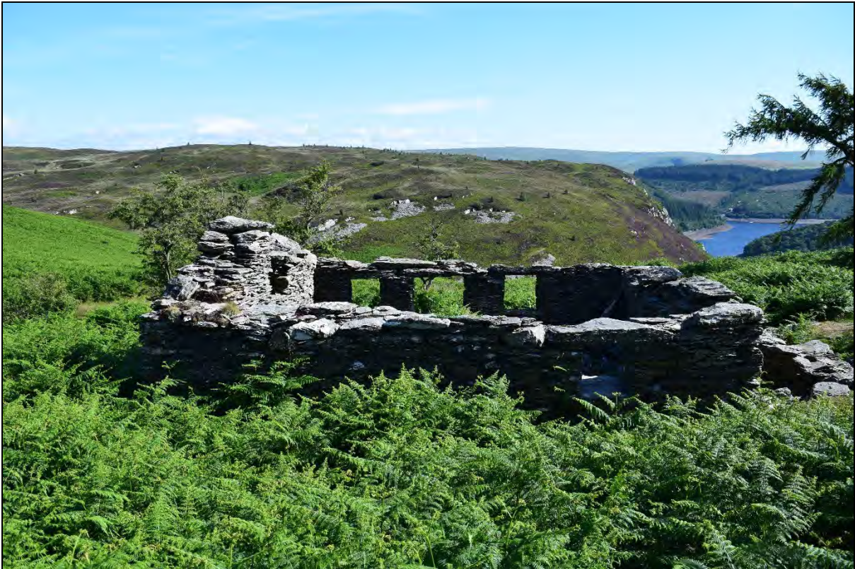
Plate 50: The ruins of Pant y Cerdin (ID number 505), close to the early 19 th century slate quarries at Nant Dolfolau. Looking south.
