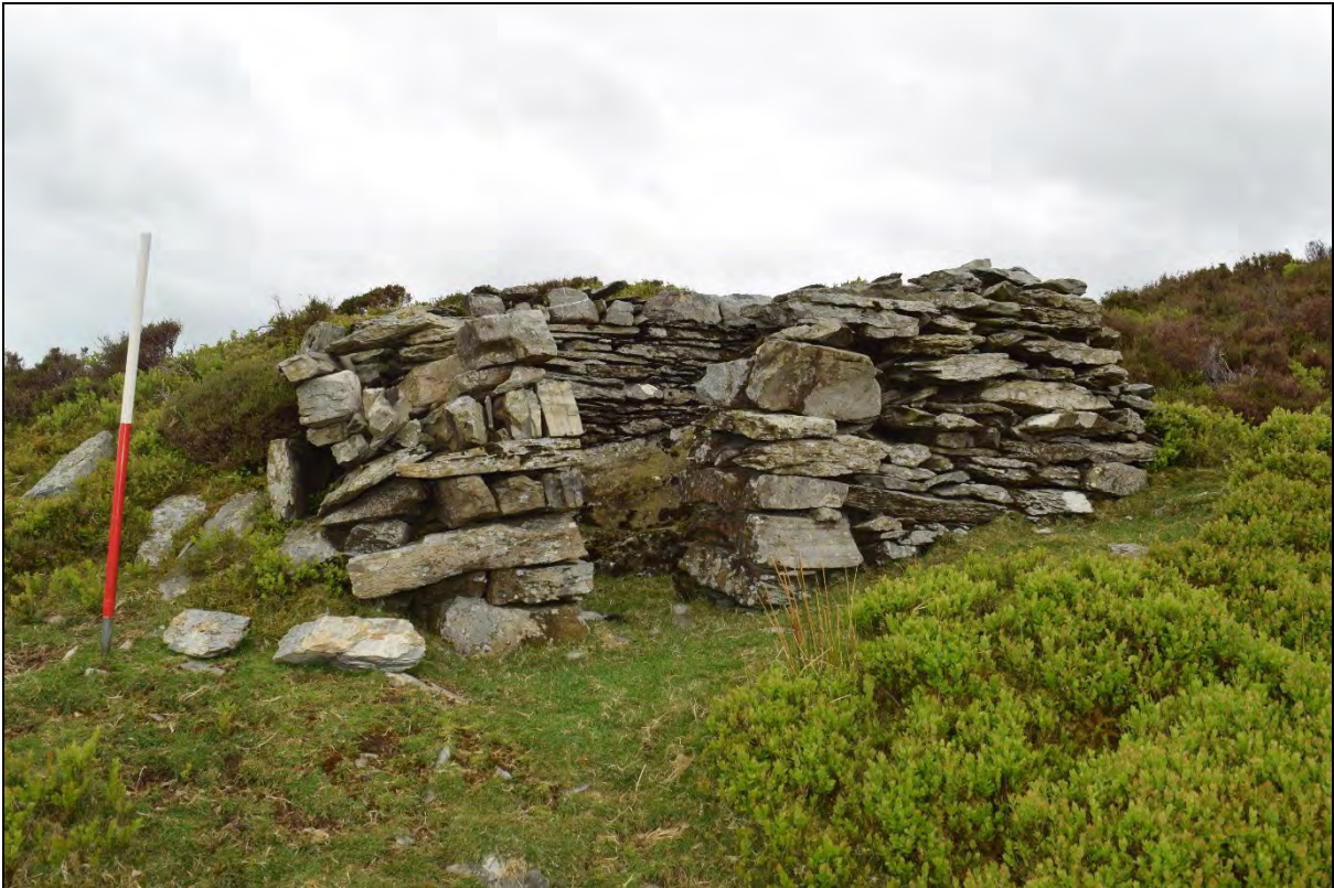
Plate 97: A stone-built Home Guard Observation Post (ID number 3217) on Cnwch, to the south-southwest of Elan Village. Looking southeast.
