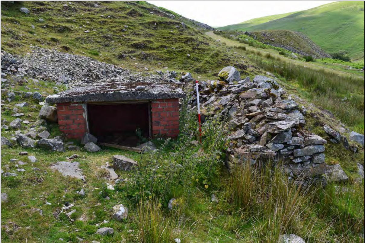
Plate 92: The explosives magazine (ID number 3325) at the Marchnant Quarry, which has a low blast wall to the right. Looking south.
