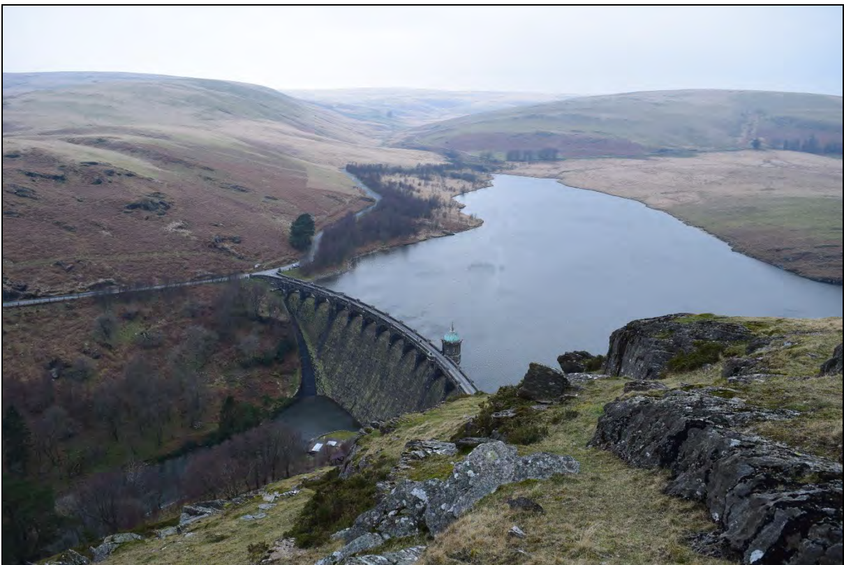
Plate 81: Craig Goch Dam, which was also completed in the early 20 th century. Looking west.
