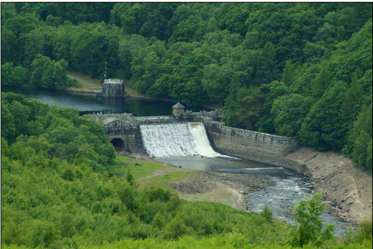
Plate 83: Dol y Mynach Dam, started in the first years of the 20 th century but abandoned at an early stage in its construction. Looking west.
