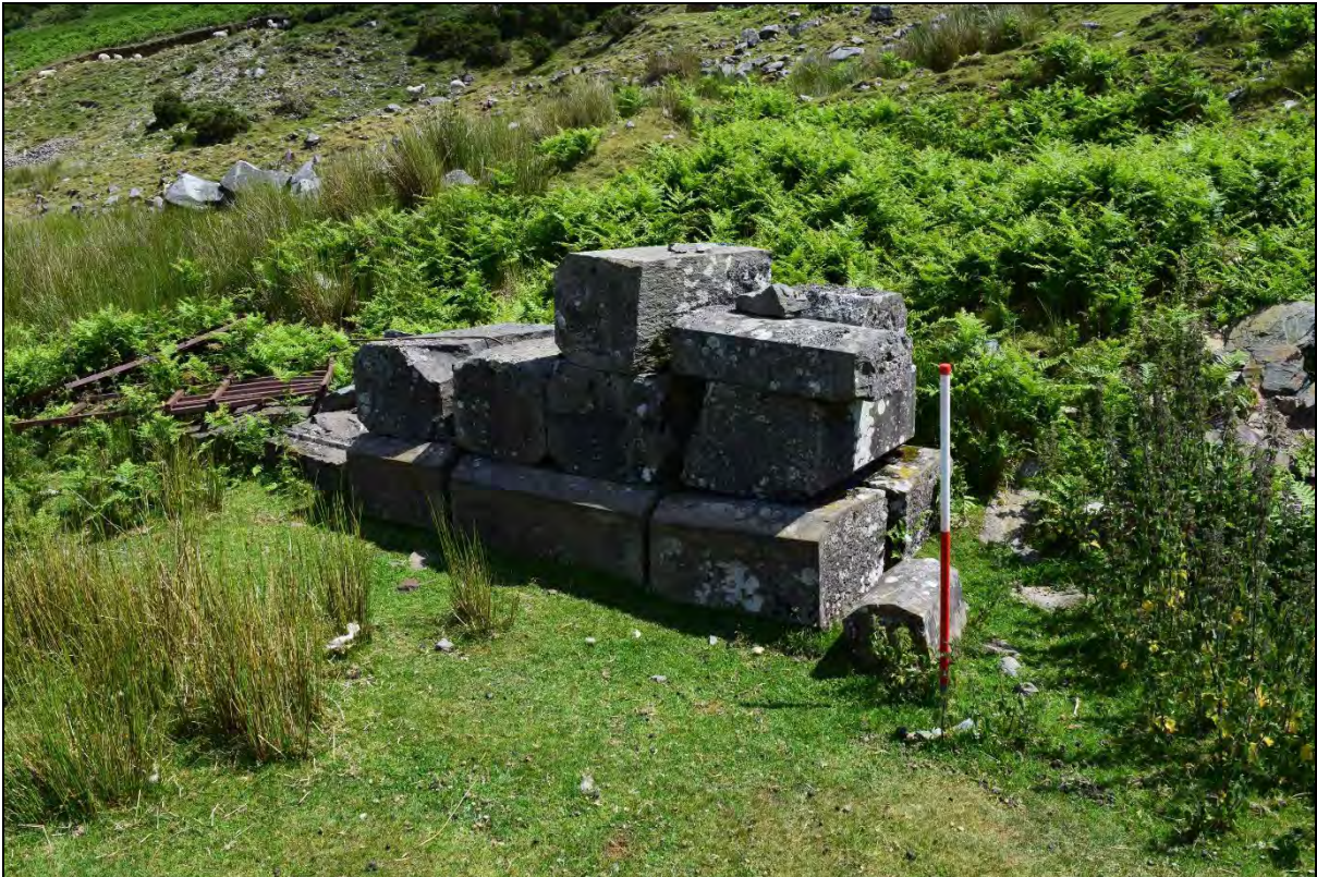
Plate 90: Dressed stones (ID number 3324) still stacked at the Marchnant Quarry which were never collected for use at the Claerwen dam. Looking east.
