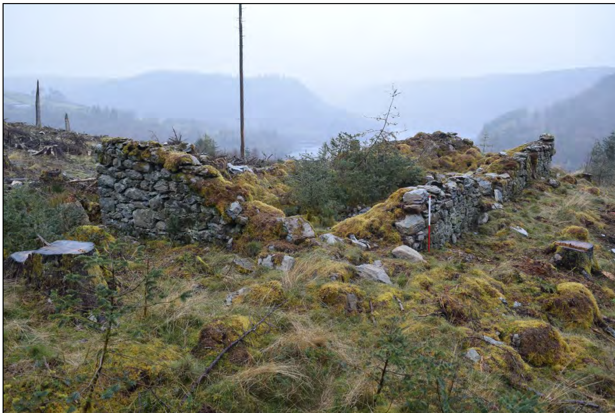
Plate 59: The Cae Sgubor Barn (ID number 362). Looking north-northeast.
