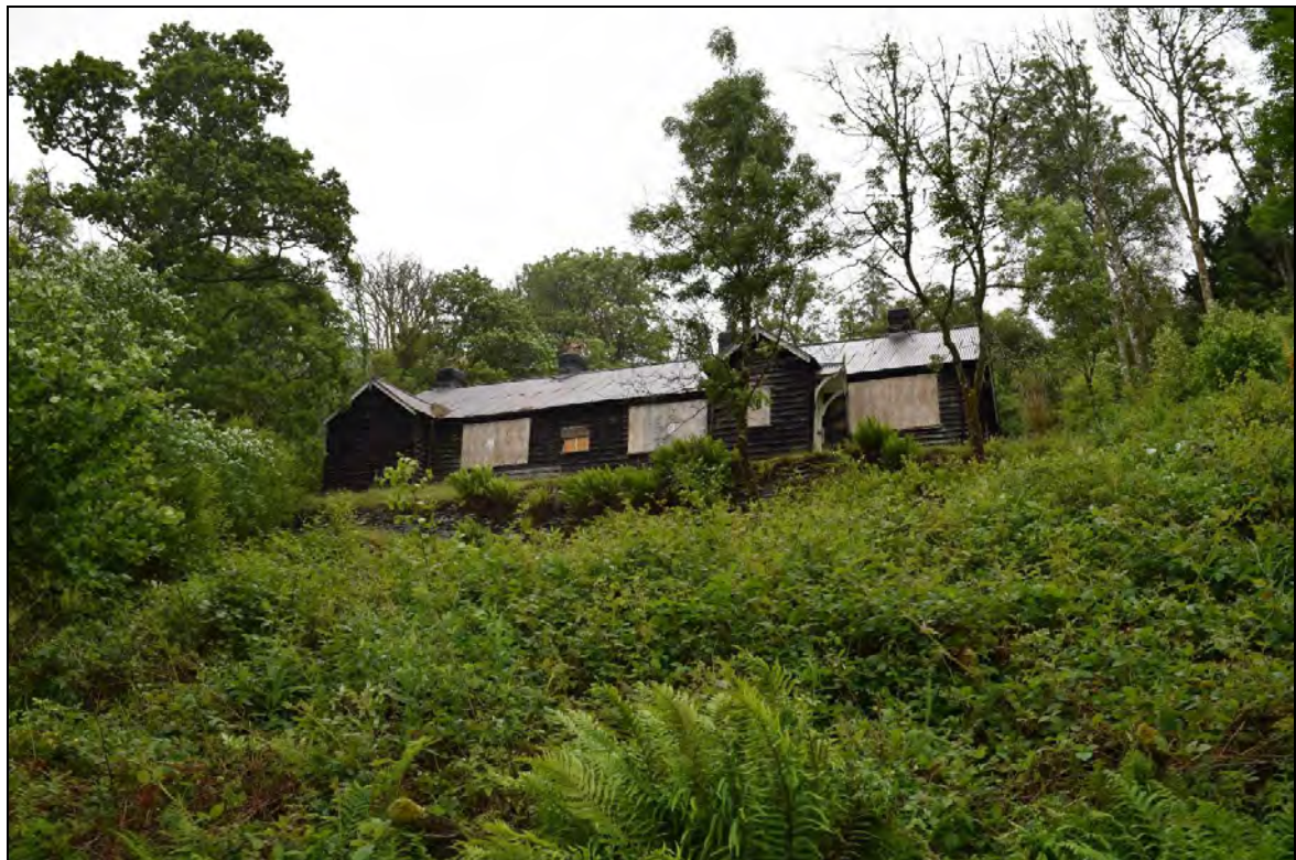
Plate 53: The Engineers House (ID number 1222) is the last of the late 19 th century Dam Builders houses and offices standing in its original position. Looking north.
