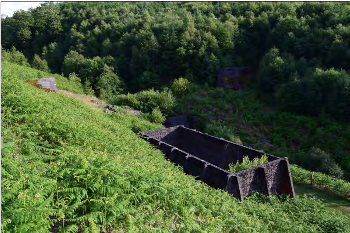
Plate 95: The site of the Nant y Gro Dam (ID number 3036) with the remains of a water tank in the foreground (ID Number 5050) . It was built to supply Elan Workers Village with water in the 1890s but blown up during military testing in 1942. Looking south.
