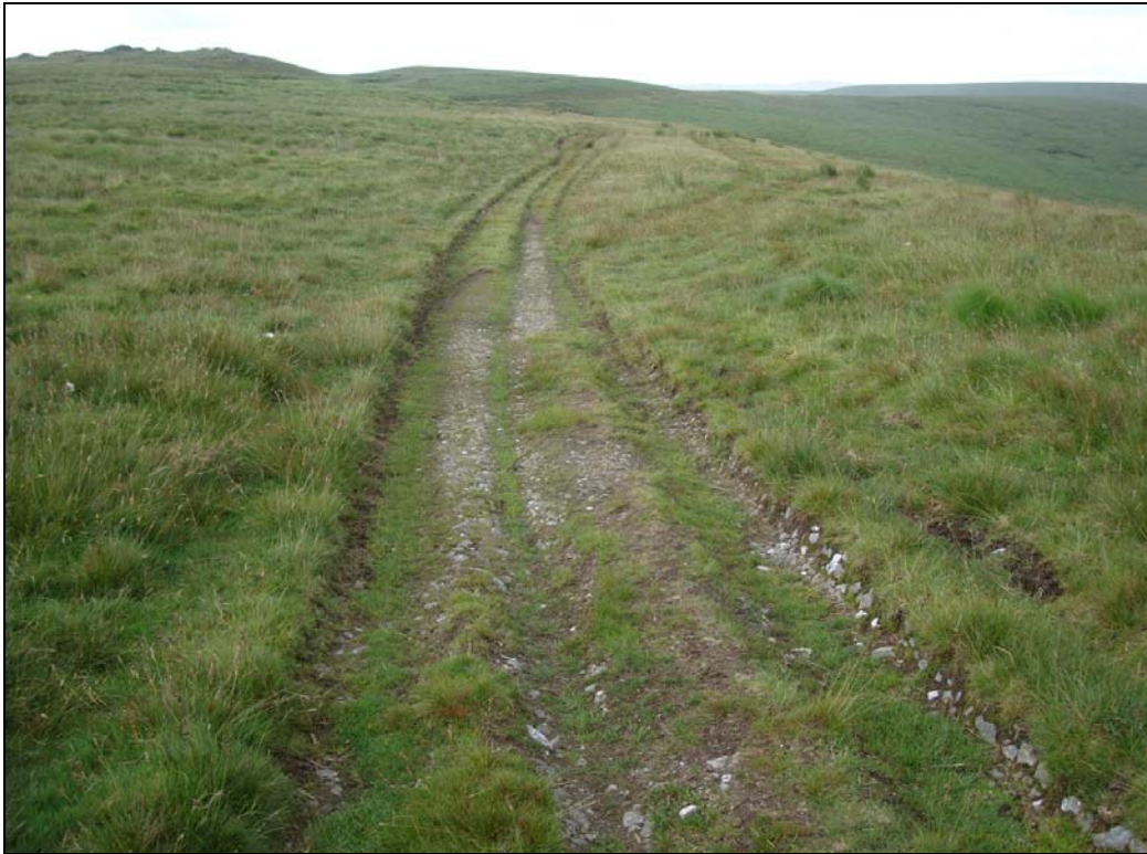
Plate 37: A photograph of a section of the Monks' Trod (NPRN 503508) showing "metalling" to the south of Llyn Cerrigllwydion Uchaf.
