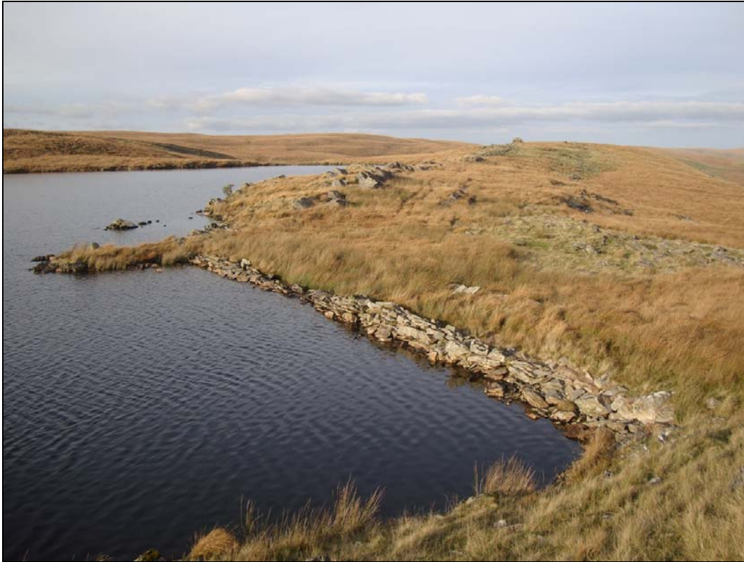
Plate 29: A photograph of the dam (NPRN 503507) at the start of the leat which took water from Llyn Cerrigllwydion Isaf lake to the Cwm Elan mine.
