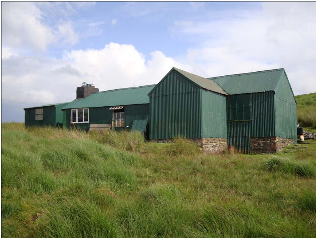
Plate 32: A photograph of the fishing lodge at Llyn Cerrigllwydion Uchaf (NPRN 503506). This corrugated iron building dates to the early 20 th century and was built by the Elan Estate.
