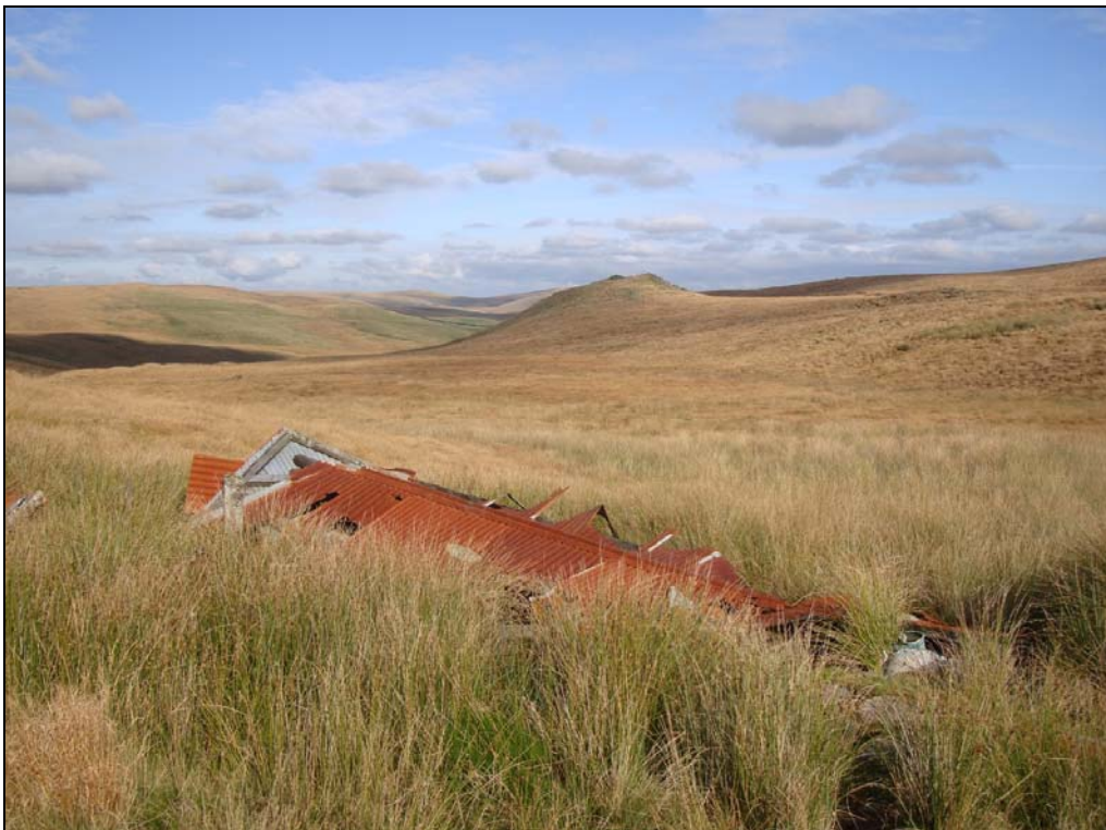
Plate 25: This photograph shows the collapsed corrugated iron shed at the site of the covered sheep dip NPRN 503527.
