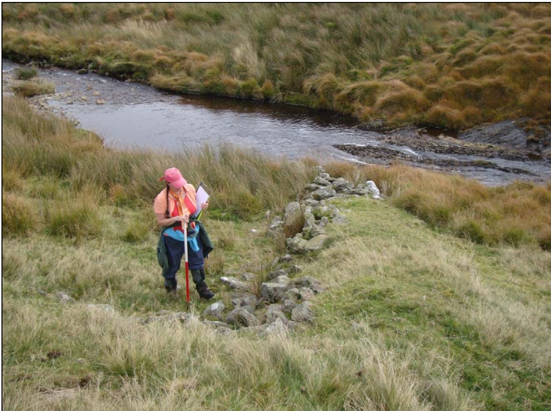
Plate 24: A photograph of the revetment wall at the sheep wash on the Nant Hirin (NPRN 503575).
