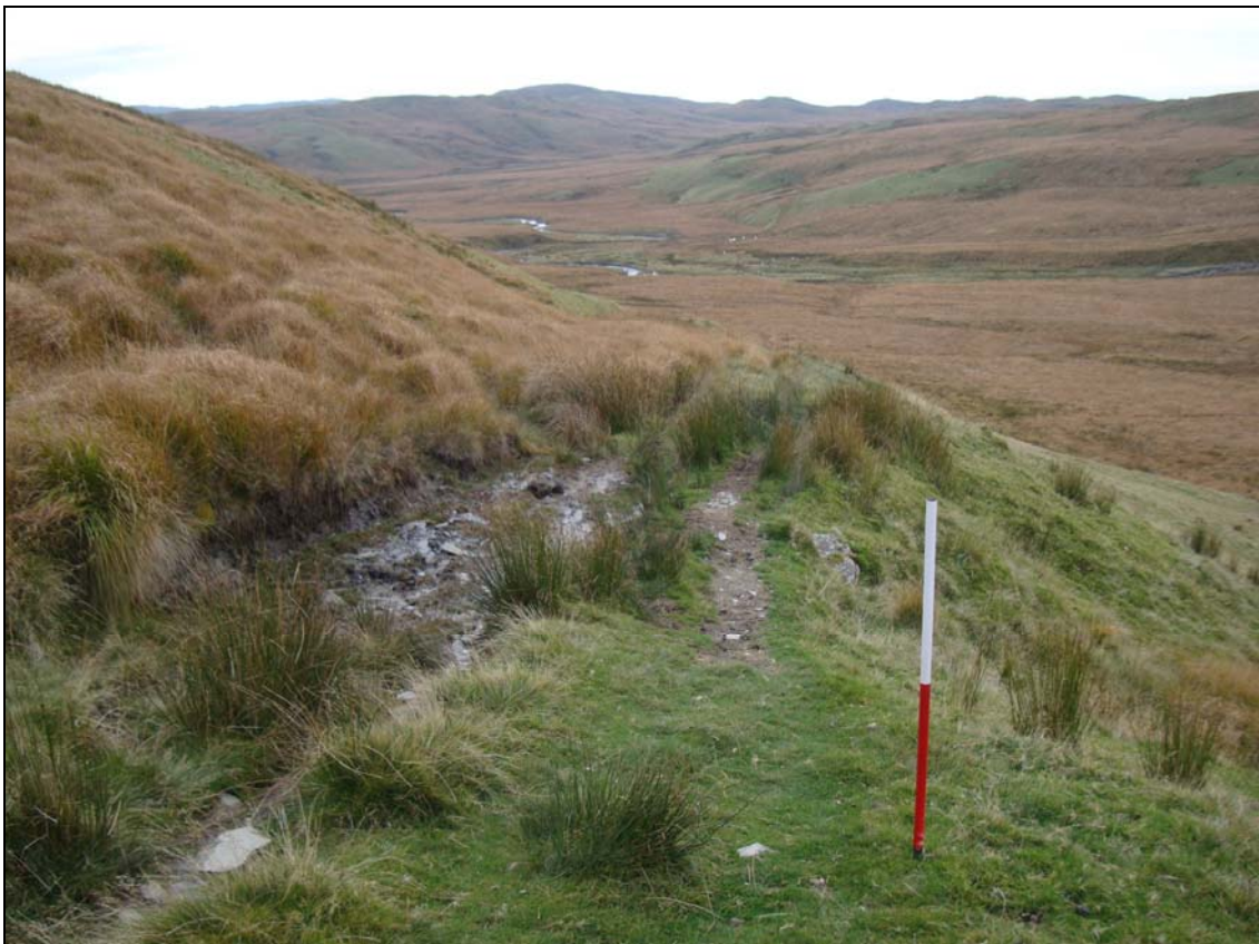
Plate 34: A photograph of an eroded “cut and fill” section of the “Monks’ Trod” on Llethr Ffos-to, looking southwest towards Rhyd Hengae.
