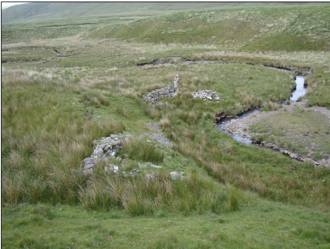
Plate 18: A photograph showing the remains of Bryn yr Ieir, where two buildings (NPRNs 503521 & 503522) have been seriously damaged by river erosion. NPRN 503522 is in the foreground.
