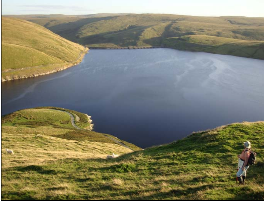
Plate 1: A photograph of the dam (NPRN 261844) at the eastern end of Claerwen reservoir, viewed from the northern side of the lake.
