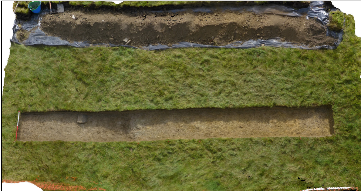
Plate 8: LAC2021_108. A vertical view of the trench taken by Ian Brooks of Engineering Archaeological Services. The dark fill (005) of the internal ditch [012] is seen to the left of centre. Looking southeast.
