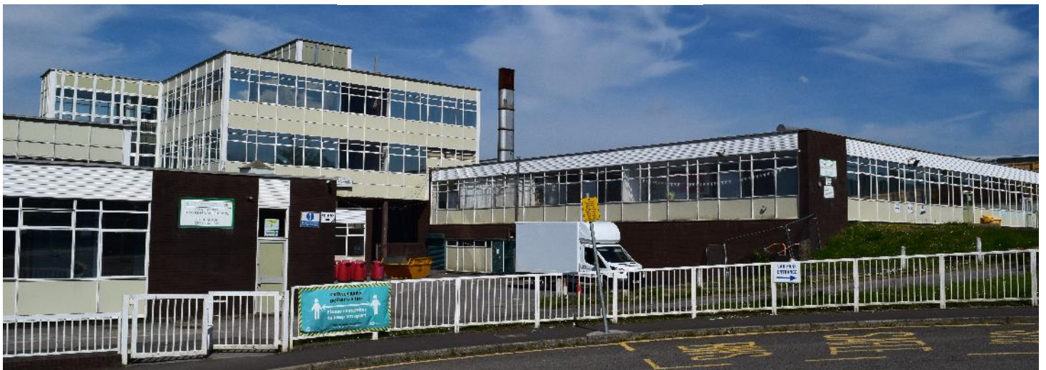
Dros yr haf fe wnaethon ni gofnod adeilad gwirfoddol o Ysgol Uwchradd Cefn Saeson, Cimla, Castell Nedd cyn iddi gael ei dymchwel. This summer we made a voluntary building recording of Cefn Saeson Comprehensive School, Cimla, Neath before demolition.
