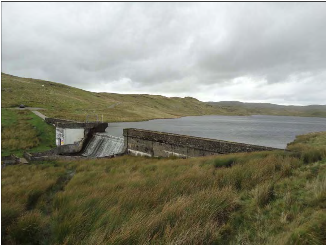
Plate 42: A photograph of the Llyn Egnant dam (NPRN 300066), looking northwest.
